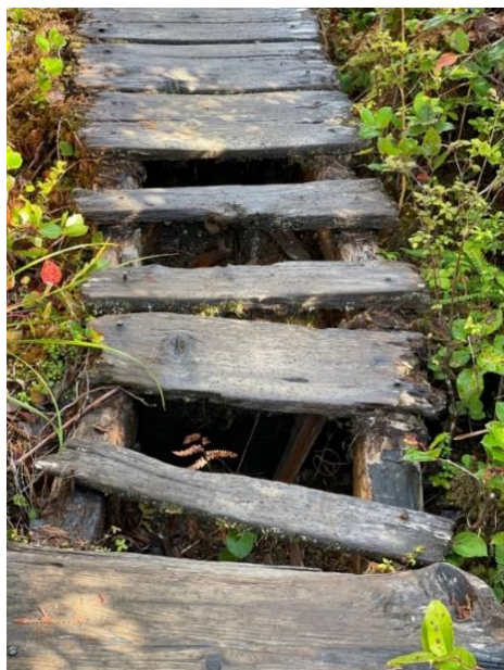
Boardwalk with broken and missing planks on parallel stringers along the Sand Point Trail
