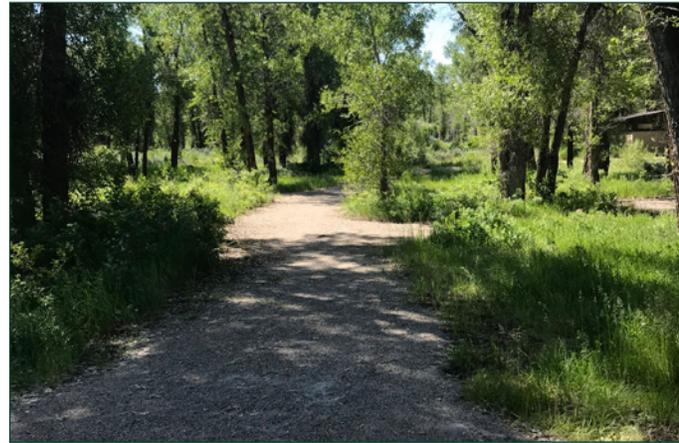
Figure 3.47 Grand Teton National Park, Wyoming, Gros Ventre Campground, six-foot-wide accessible crusher fine aggregate.
