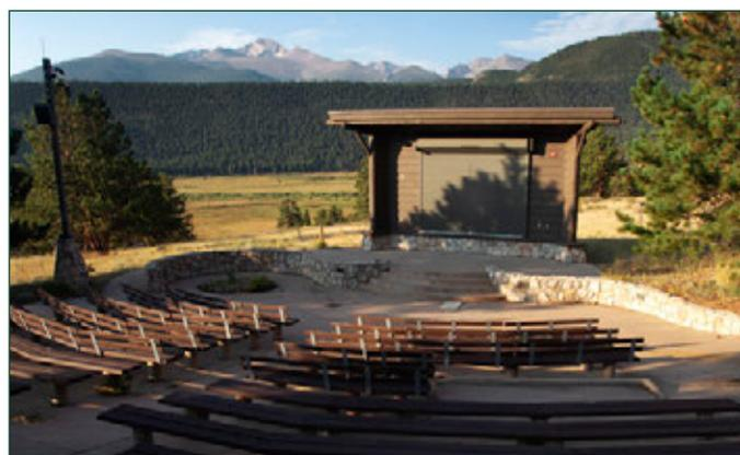
Figure 3.108 The “after” image of the same amphitheater updated technology and provides accessibility to 50% of seating, including 10 wheelchair spaces integrated throughout. Seating includes benches with and without backs to enhance comfort and usability for all visitors.
