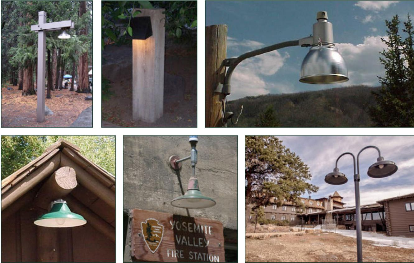
Figure 3.102 Captions ordered left to right, top to bottom: Rustic wood frame lighting post at Yosemite National Park campsite; Wedge bollard light to brighten walkways at Yosemite National Park; Sky guard lighting fixture at Yellowstone National Park; Light on A-frame structure at Yellowstone National Park; Industrial shaded light at Yosemite National Park; Tall light posts at Grand Canyon National Park’s Historic District.
