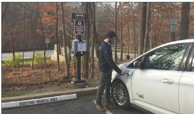
Figure 3.129 Example of Electrical vehicle charger installed at Catoctin Mountain Park, Maryland. Charger installation requires a transformer that can accommodate the charging stations. This may require a new transformer, new panel, new disconnect switch, meters, bollards, electric vehicle parking signs and striping, electrical conduits, and the charging stations themselves.
