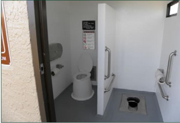
Figure 3.87 Squat toilet adjacent to a standard toilet riser allows users with different preferences to have options.
