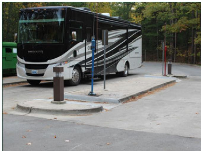
Figure 3.125 Sleeping Bear Dunes National Lakeshore, Michigan, Platte River. Campground dump station includes an accessible RV parking lane with island access aisle to approach station components.
