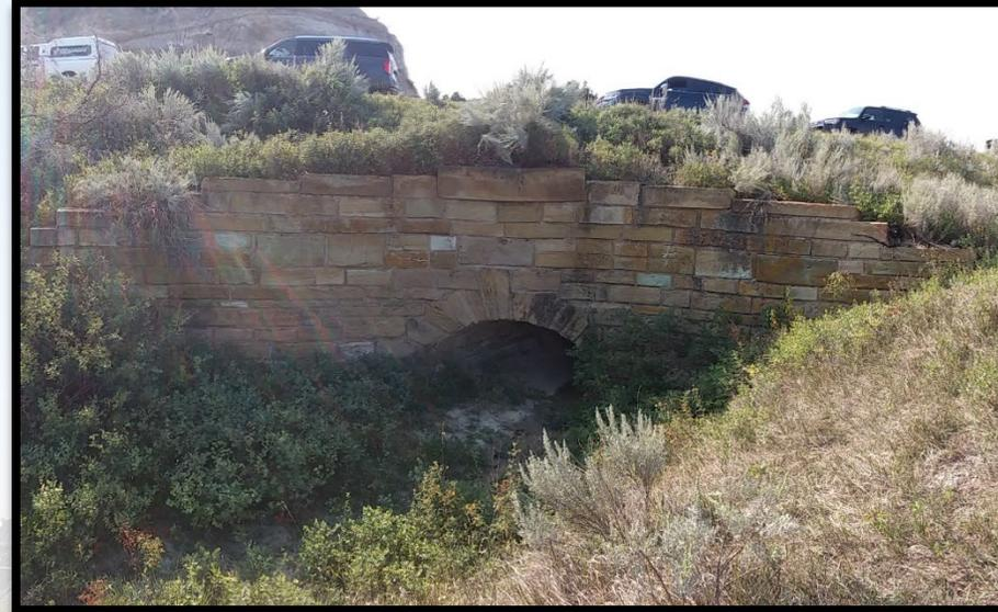
Example of stone arch culvert that would be repaired during proposed replacement (remove sediment, repoint the mortar, replace fallen stones).
