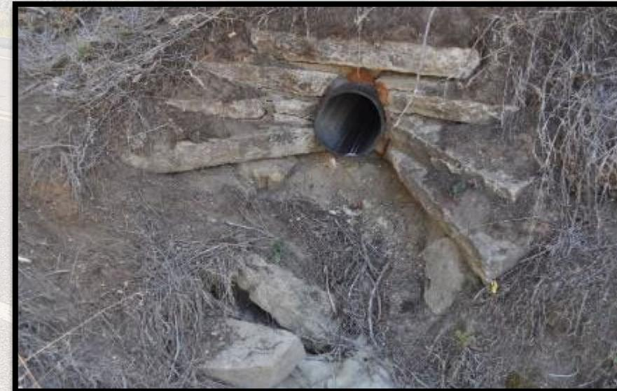
Example of pipe culvert to be replaced. This culvert is too small to allow for appropriate drainage and would be replaced with a larger concrete pipe.
