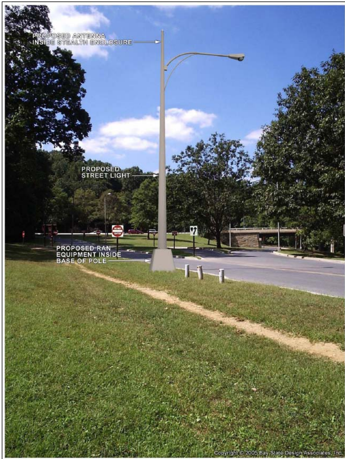
Figure 38: Crown Castle – Typical DAS Installation
