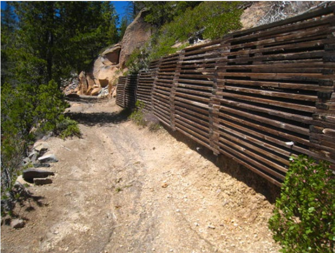
Figure 1. Undercut retaining wall and trail tread loss.
