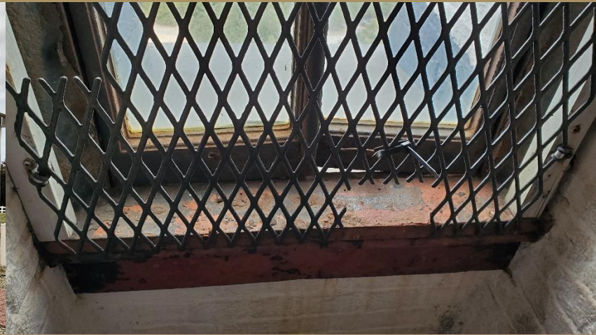
Grates installed over some windows
