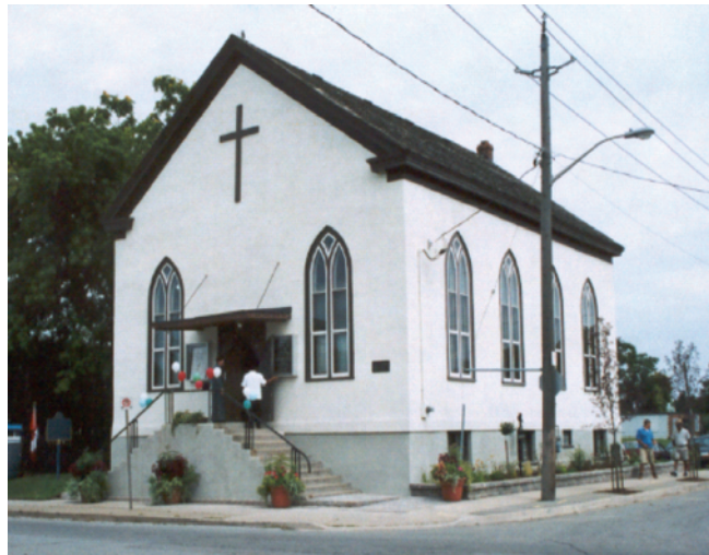
Figure 2-12. BME Church, St. Catharines, Ontario, the church at which Harriet Tubman worshipped, now a Canadian national landmark for its association with Tubman.
