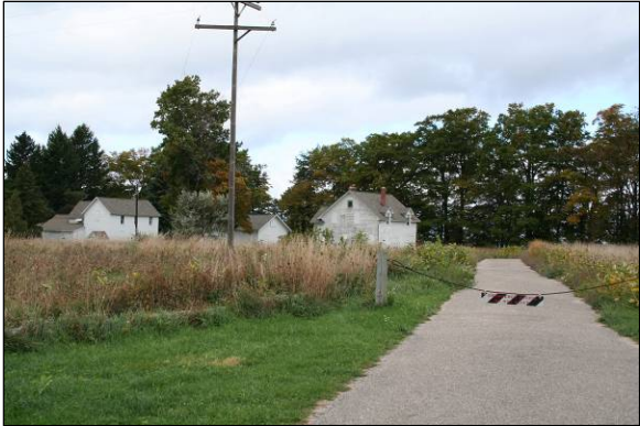
Burfiend (west) driveway and parking area (MBD 2005)
