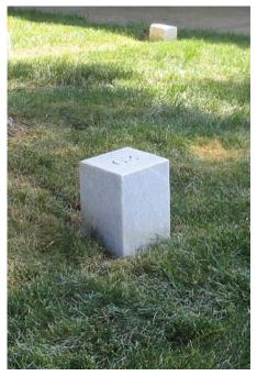
Figure 4.13: Reproduction Civil War-style block at Seven Pines National Cemetery. The font used for the grave number does not match the historic font; in addition, this block was installed at approximately 10" high, while historically the blocks were installed at 6" (historic block in background). SUNY ESF, 2006.
