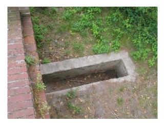
Figure 4.8 (left): Flooding in Division A along south side of inclosure wall related to inadequate grade and drainage through the wall. SUNY ESF, 2006.
