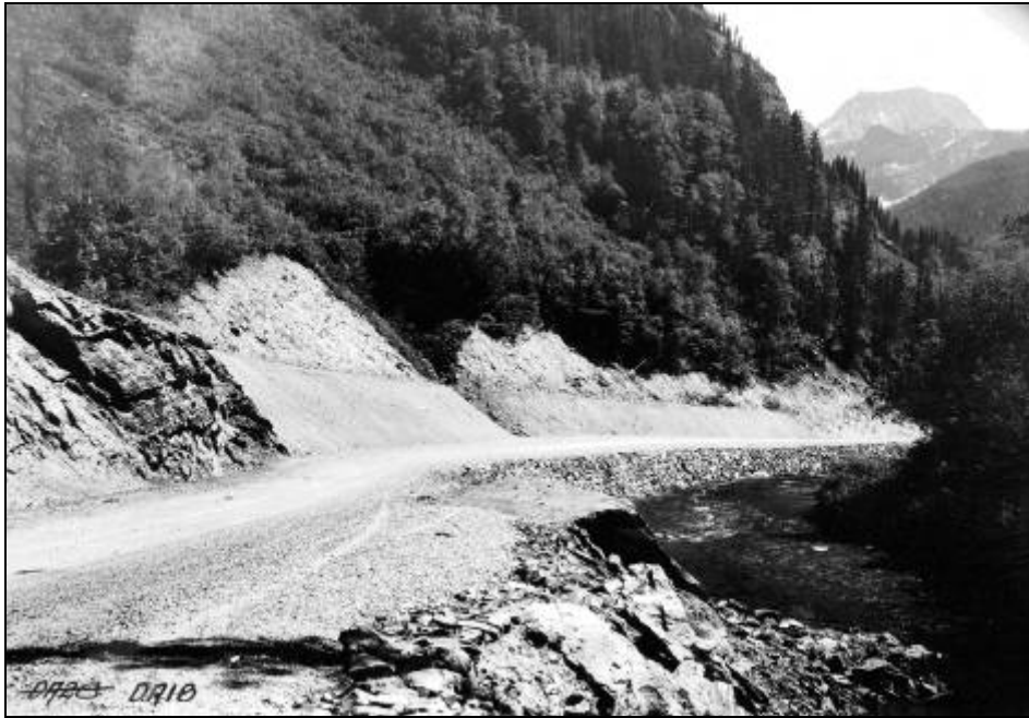
Photo 3. McDonald Creek bank stabilization with riprap along the Going-to-the-Sun Road, 1934 (GNP Digital Image Database Accession Number 11616)
