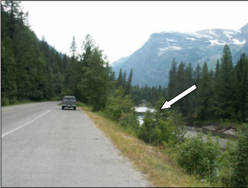
Photo 2. View of McDonald Creek bank stabilization site to visitors traveling west. (View is from pullout approximately two-tenths of a mile above site.)
