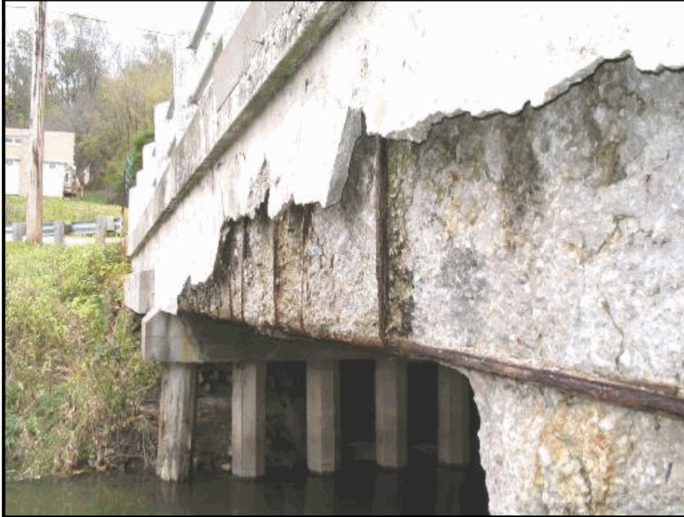
*Figure 3: The concrete girder of the Waste Weir Bridge has deteriorated to the point where steel rebar is now exposed.*
