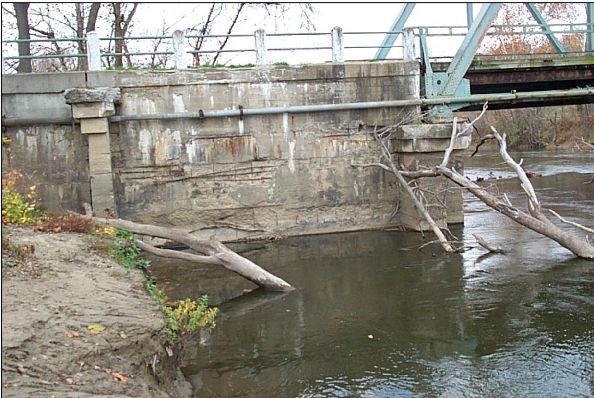
*Figure 2: The southern abutment shows a moderate degree of scour from the River, and exposed steel rebar.*
