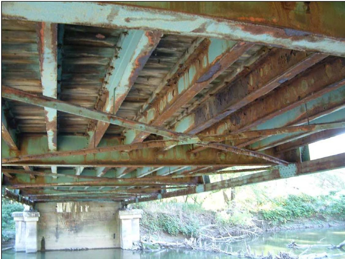
*Figure 1: The underside of Fitzwater Truss Bridge is severely rusted and deteriorating*
