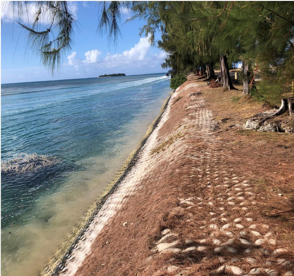
EXAMPLE OF SEDIMENT WASHOUT DUE TO BOAT WAKE
