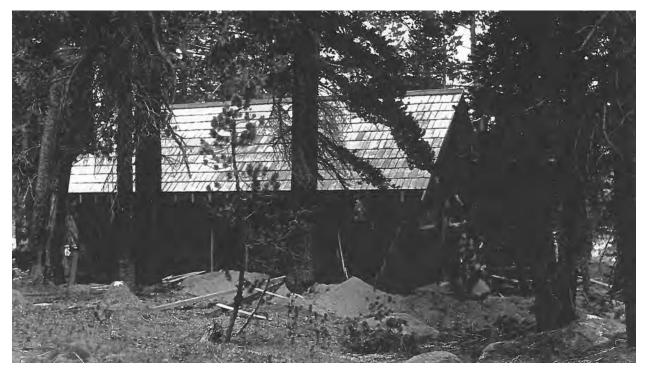
Figure 2-17. Comfort Station (CS3024) under construction in 1932. The building was one of several designed in the park rustic style by the NPS Western Field Office (source: YOSE 1932 Superintendent's Report).
