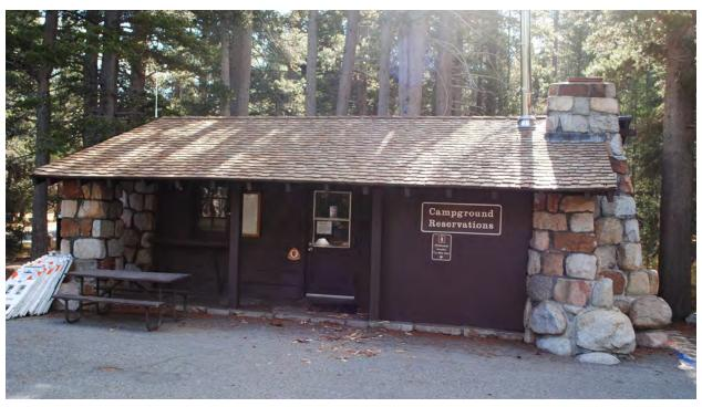
Figure 3-70. Porch extending the full width of the front elevation (source: Mundus Bishop, 2019).
