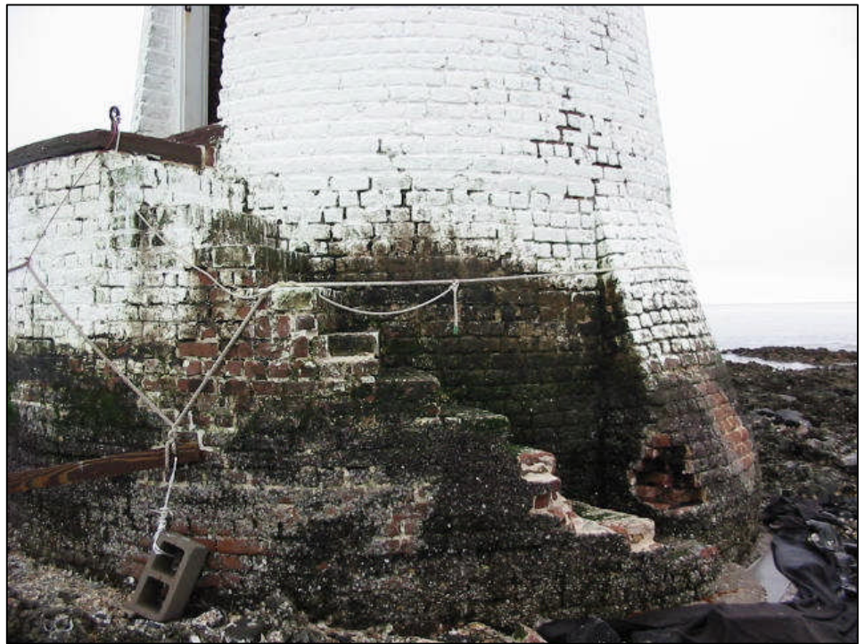
The NPS has been making emergency repairs to the lighthouse's exposed wooden foundation that is being damaged by shipworms.
