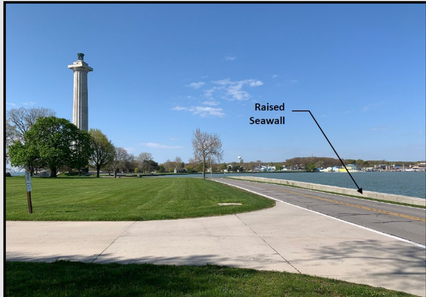
Visual Assessment of the Raised Seawall
