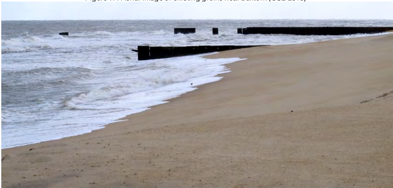
Figure 18. Ground photo looking south at two of the groins at the former location of the Cape Hatteras Lighthouse. The structures extend into the ocean from right to left and are constructed of pre-cast concrete sheet piles linked by timber whalers. Some sheets have collapsed or washed out as indicated by the gaps in the structure along the top edge of the image. (Image credit: CSE, November 4, 2013)
