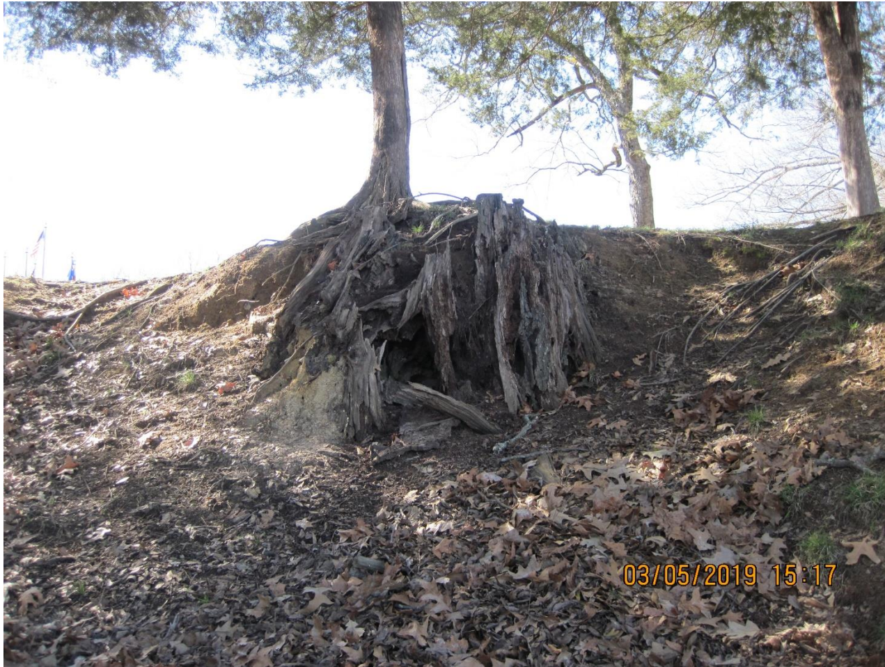
Figure 12 Close-up of erosion undermining tree from Fig. 10
