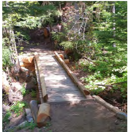
Figure 7. An example of a recently built puncheon bridge on the Thunder Creek Trail
