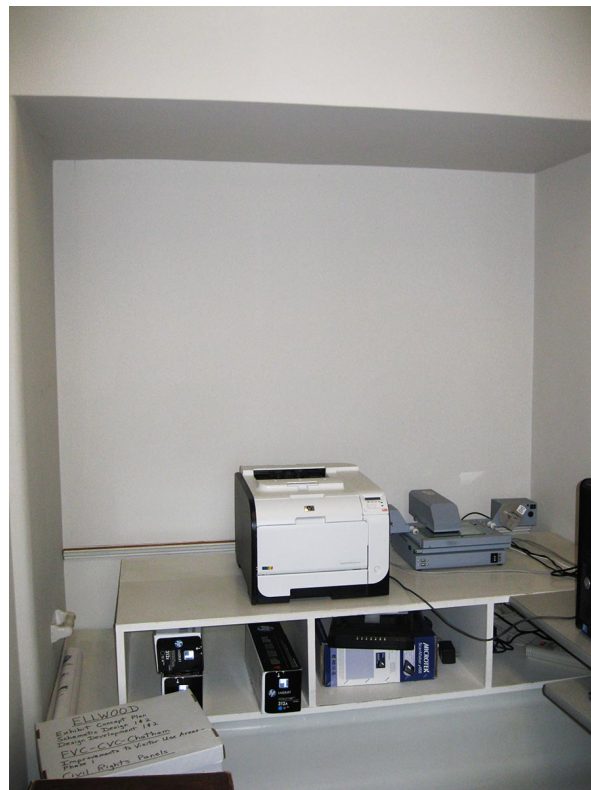
Inside the former bathroom on the second floor of Chatham Manor. The bathtub is visible below the makeshift cabinets holding office equipment. A wood support will be built over the bathtub and the air handler will be placed on the platform. The ductwork will vent through a hole cut in the plywood ceiling above.
