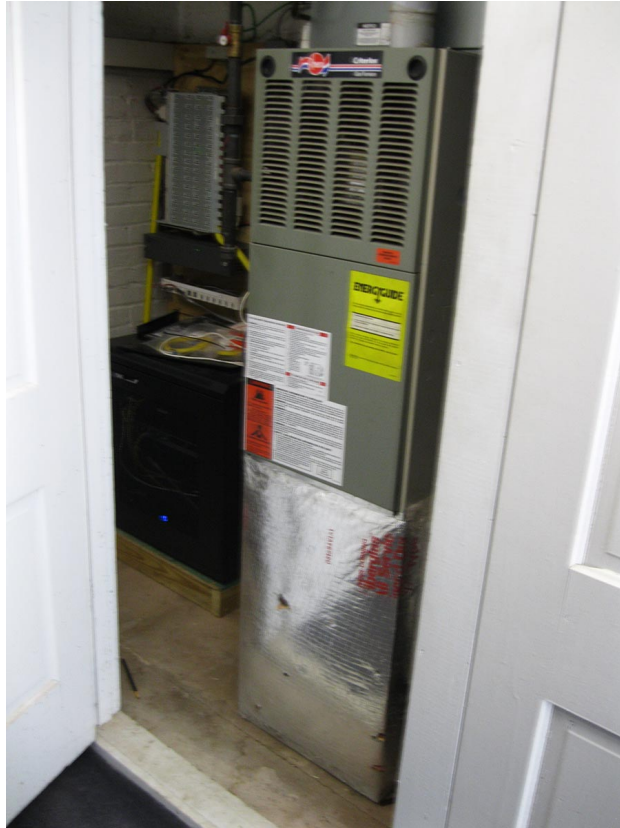
Air handler inside the Chatham Carriage House, located inside a closet. The handler will be replaced.
