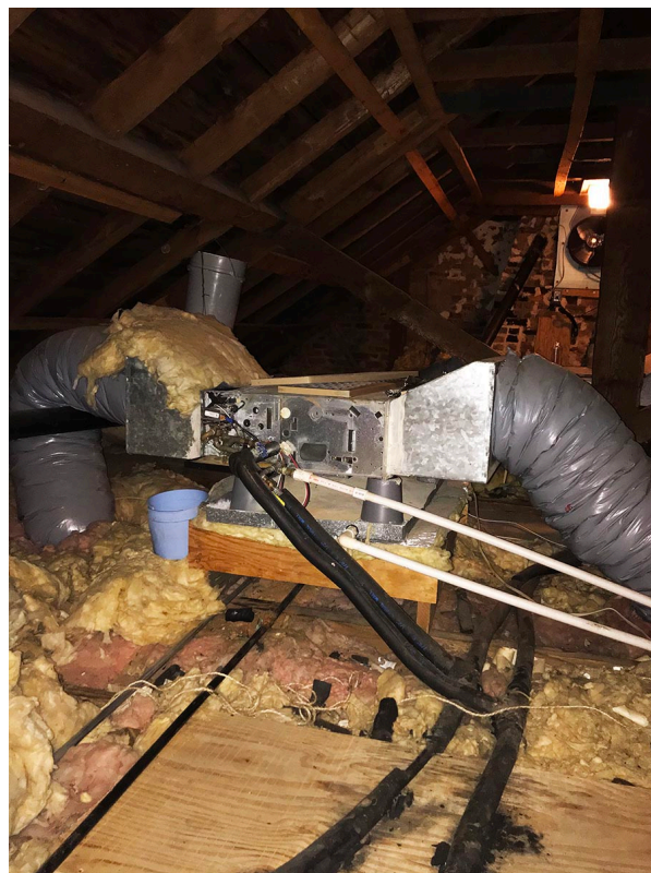
One of seven chiller units in the attic of Chatham Manor. The units will be removed
