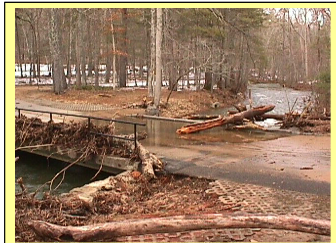
Figure 3.4-2. Debris at the Otter Creek Bridge Site Following a Major Storm
