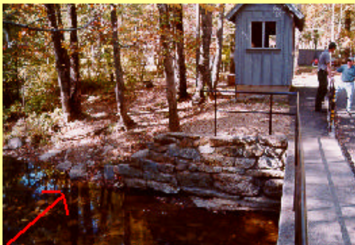
Figure 1.3-3. Damage to the Otter Bridge Abutments
