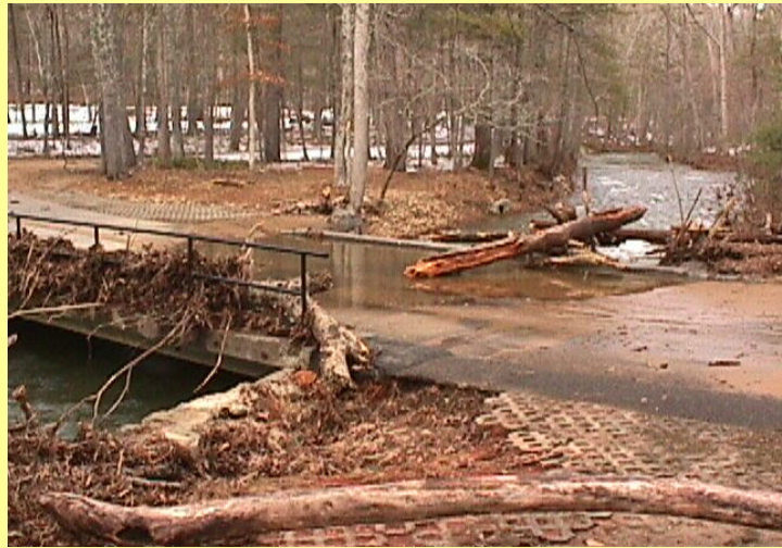
Figure 1.3-1. Debris Jam and Flood Damage at Otter Creek Bridge During a Recent Rain Event
