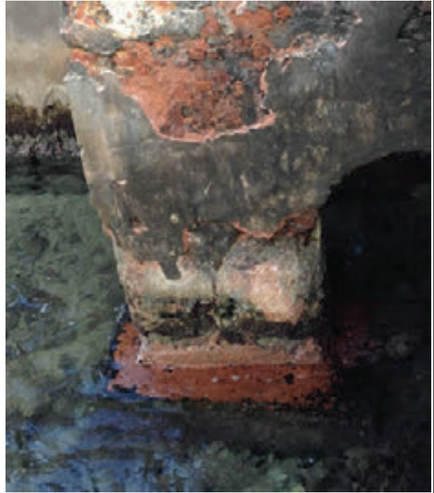
Photo 26: Erosion at base of House 2's support.
