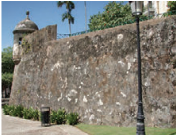
Photo 3: East Section, small percentage of inappropriate repair and vegetative removal.
