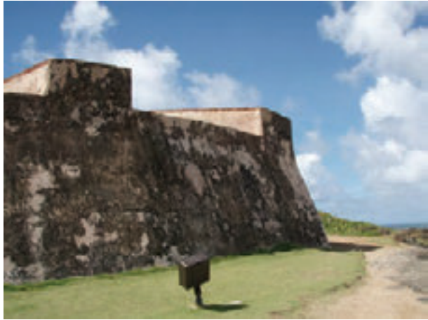
Photo 1: East Exterior (showing black fungus and deterioration).
