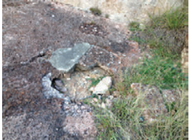
Photo 22: Close-up of hole above cistern #1
