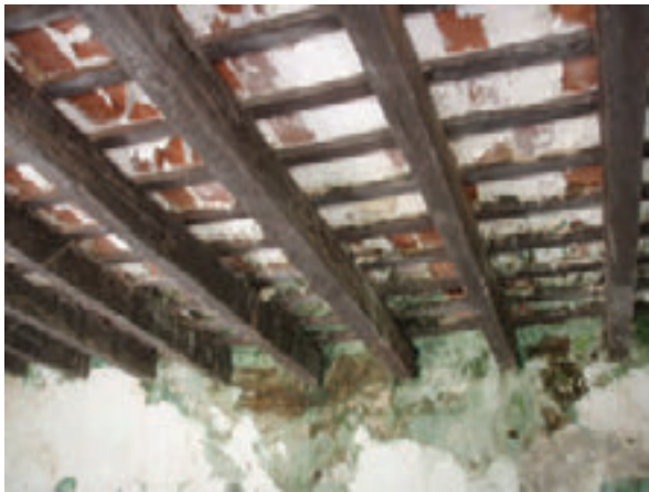
Photo 11: Replace/Reset sagging beams in forecourt house.
