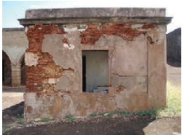
Photo 2: Applications of Portland cement advancing the deterioration of the exterior walls of the house on the forecourt.
