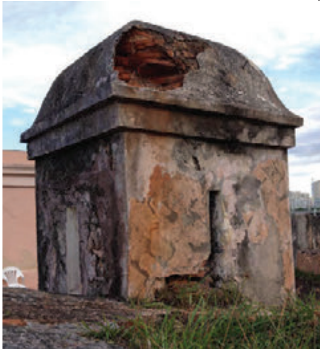
Photo 35: Missing blocks from sentry box roof.
