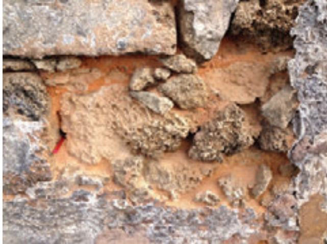
Photo 15: Example of cavities in exterior wall and missing bricks/stone.
