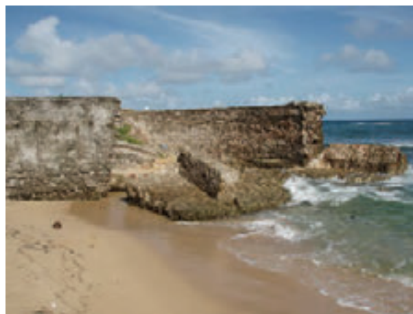
Photo 2: Northeast corner has fallen on exterior side and split into pieces.
