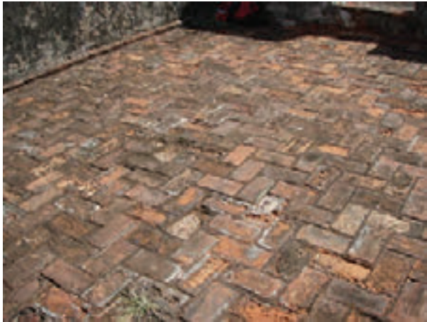
Photo 3: Brick roofing has weathered and deteriorated significantly on all brick roofs.
