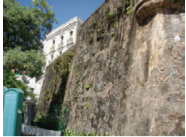
Photo 2: Central section needing vegetation and inappropriate repair removal.
