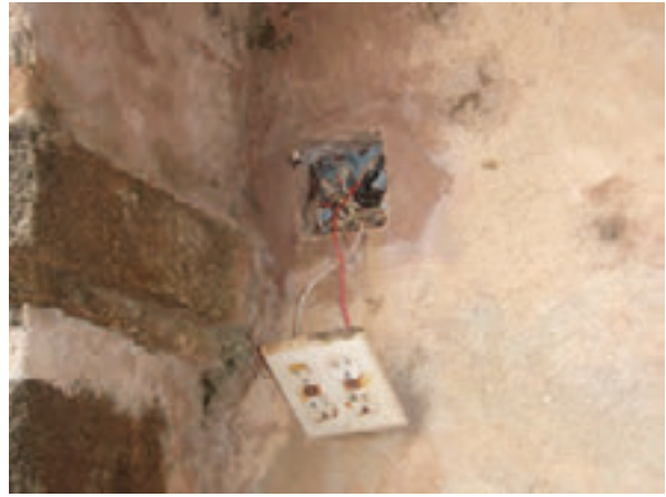
Photo 10: Replace deteriorated electrical components.
