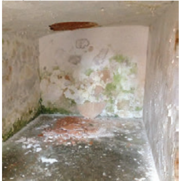
Photo 24: Ceiling coating delaminating in Room 7, pulling off parts of brick with it.
