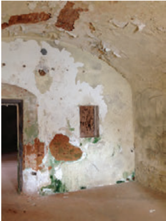
Photo 23: Paint and other coatings peeling off walls and ceiling in Room 1.
