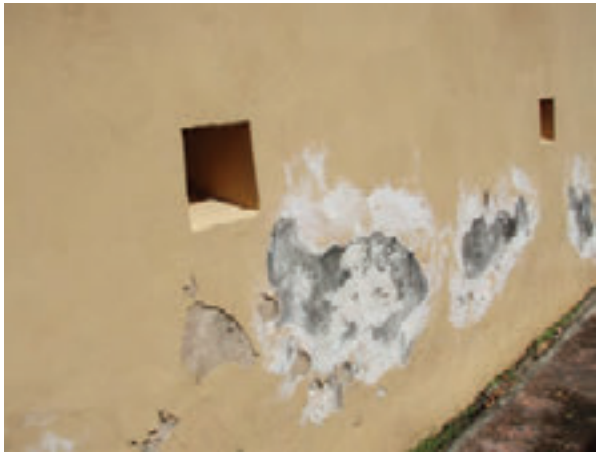
Photo 1: Continued application of inappropriate repair material and paint further deteriorates walls and promotes fungal growth.
