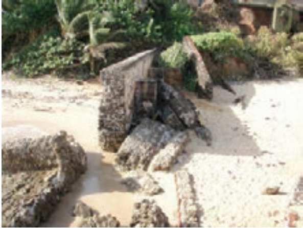
Photo 3: East exterior still standing, approximately 20' long section closest to street is lying on its side underneath the sand.
