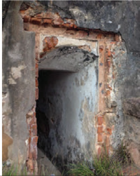
Photo 16: Close up of typical cement and mortar erosion.
