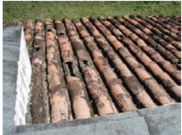
Photo 4: Deteriorated roof tiles
