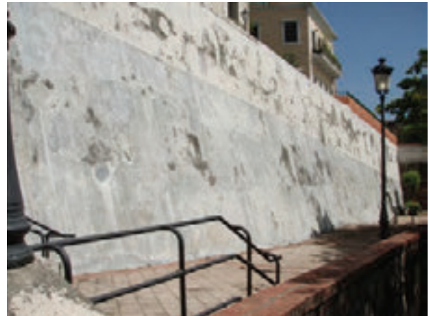
Photo 4: West section that has been covered with a mixture of lime and concrete. Dark spots indicate trapped moisture and fungal growth from underneath.
