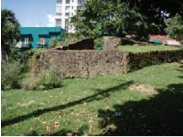
Photo 1: Front view of battery, east exterior, remove vegetation, repair walls and resurface.
