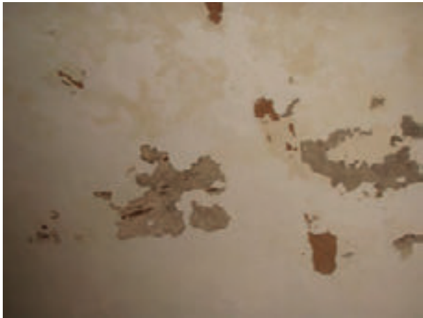
Photo 5: Remove inappropriate paint and repairs to properly apply limestone plaster.
