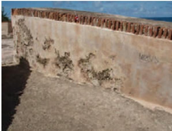
Photo 3: Deteriorating embrasure walls and brick cornering.
