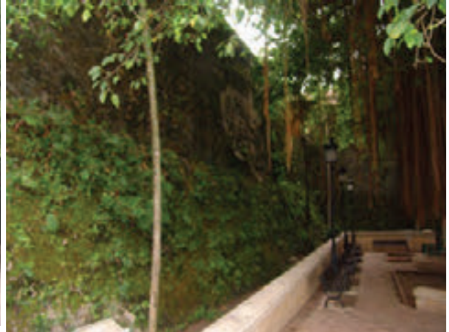
Photo 2: Significant vegetation and removal of inappropriate repairs needed.
