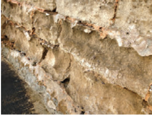
Photo 37: Typical erosion of sandstone courses along the base of the Fort.
