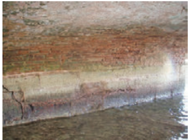
Photo 6: Cracking/erosion of bridge support structure.
