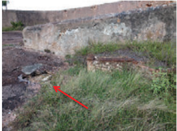
Photo 20: Hole developing above cistern #1 in the forecourt (shown also ramp retaining wall and planter).
