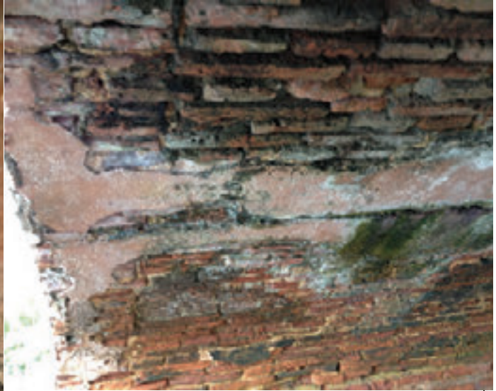
Photo 6: Efflorescence associated with crack.
