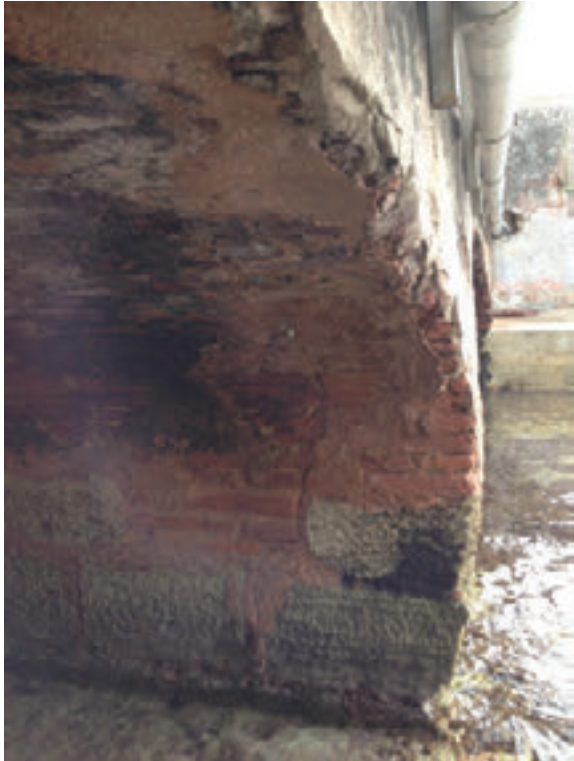
Photo 7: Bulging arch support with vertical crack.
