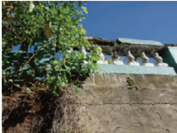
Photo 3: Deteriorated Concrete railing
