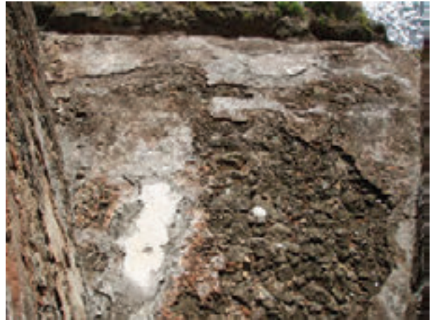
Photo 4: All walls and floor surfaces have inappropriate repairs or their surfaces have been completely eroded to substrate.
