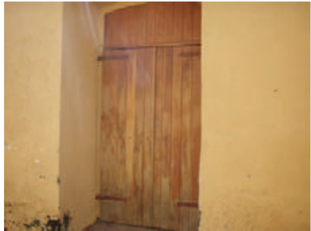
Photo 6: Refinish exterior doors and window frames.
