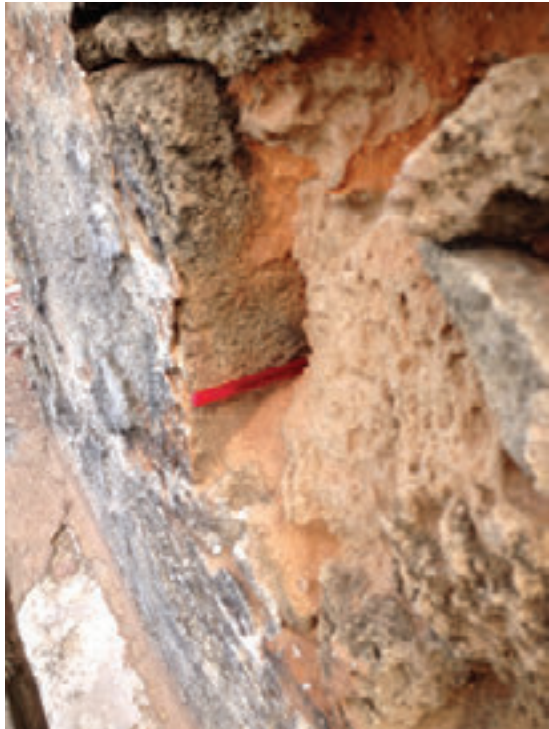
Photo 19: Voids six inches deep into wall.
