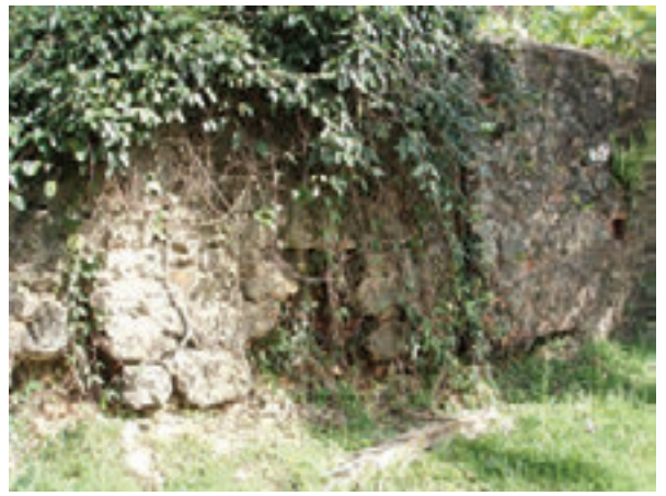
Photo 4: South Exterior wall overgrown and foundation has completely fallen away in places.
