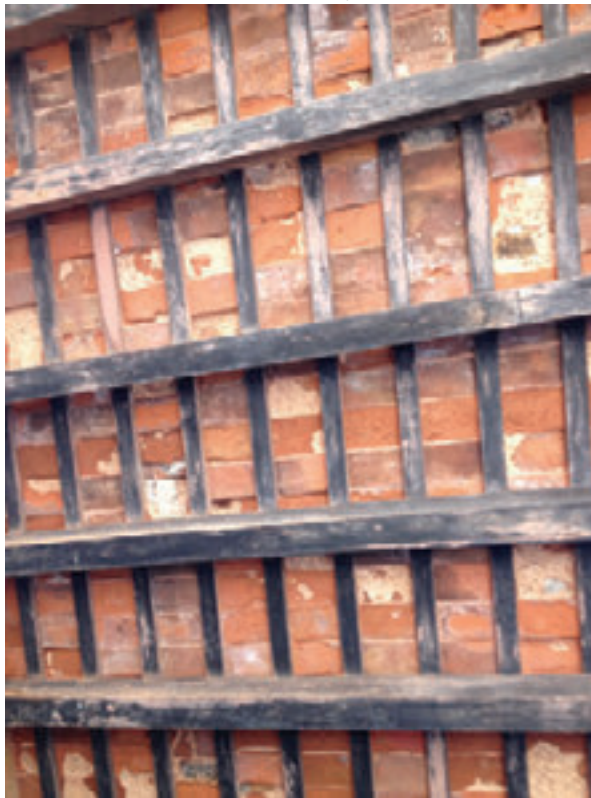
Photo 11: Portico roof bricks, eroded.
