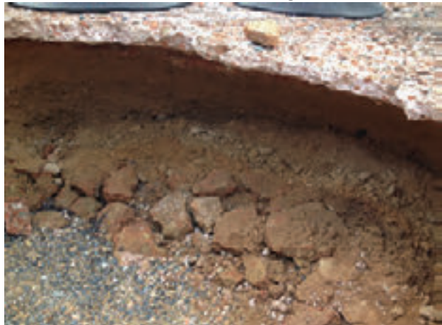
Photo 4: View of void undercutting deck.
