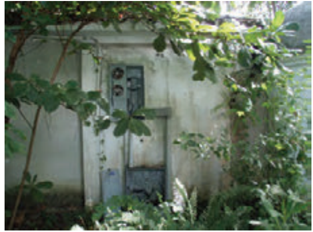
Photo 2: Gutted electrical service
