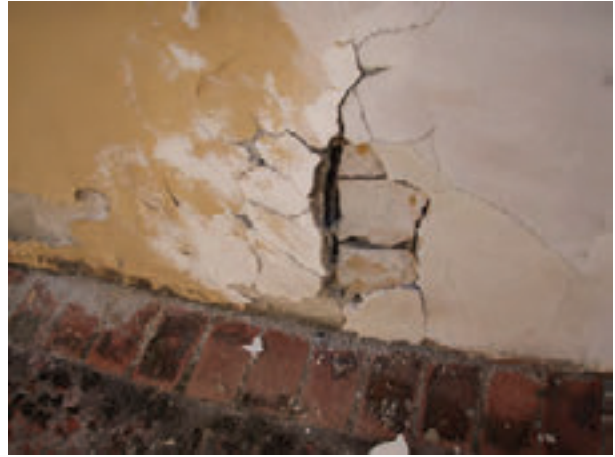
Photo 4: West exterior wall damaged from installation of light panel box on interior of west entrance.
