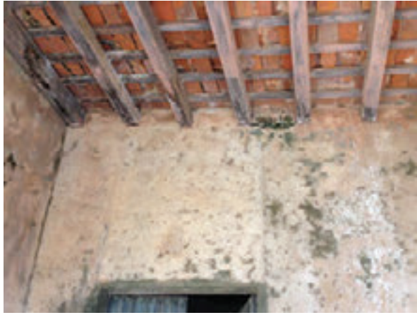
Photo 11: Portico roof bricks, eroded.
