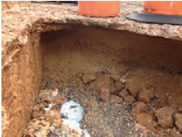
Photo 3: Depth of bridge deck void.
