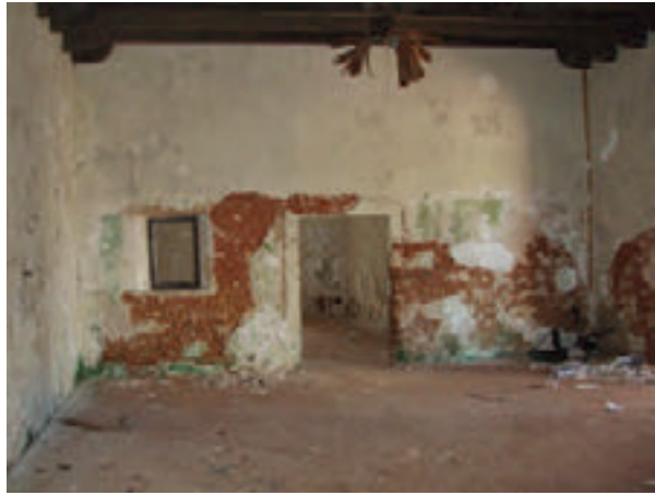
Photo 1: Inappropriate paint and repairs has caused larger sections of plaster to fail.
