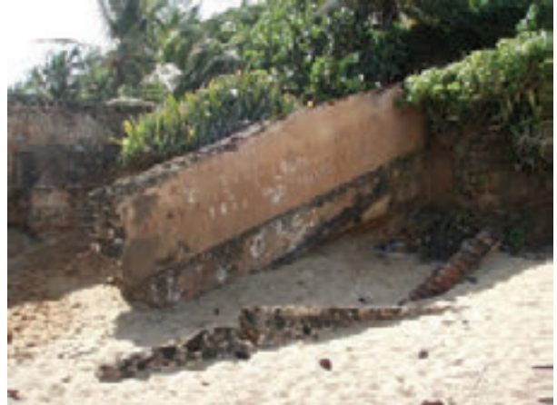
Photo 4: Possible interior or west exterior wall that has been displaced, now located south towards street.
