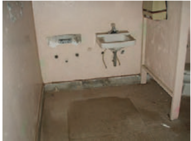
Photo 6: Deteriorated plumbing fixtures.
