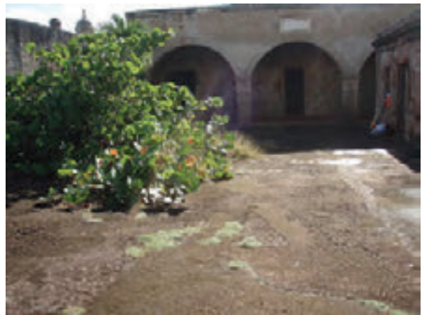
Photo 8: Remove vegetation from Fort, remove inappropriate repairs and resurface uneven floors.
