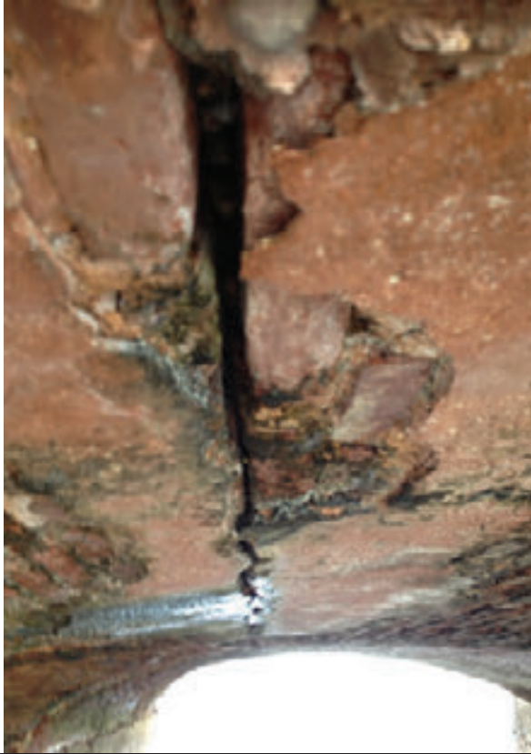
Photo 7: Bulging arch support with vertical crack.
