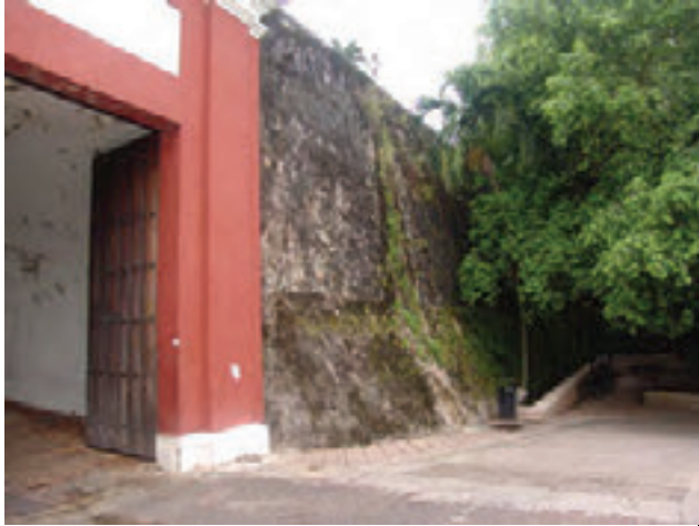
Photo 1: Significant vegetation and removal of inappropriate repairs needed.
