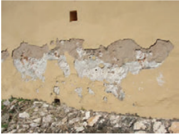
Photo 3: Remove inappropriate paint and repairs to properly apply limestone plaster.
