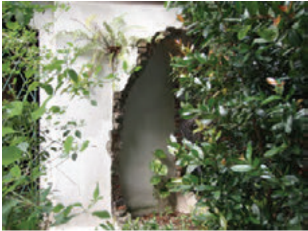
Photo 1: Demolished northwest sentry post with opening bricked up with CMU.
