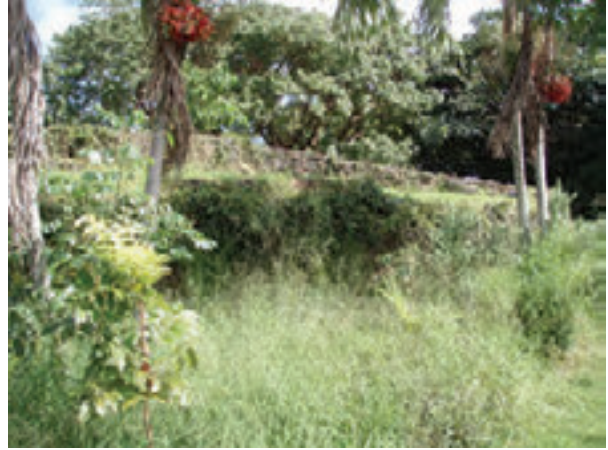
Photo 2: South exterior is completely overgrown, remove vegetation, repair walls and resurface.
