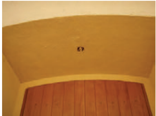
Photo 2: Previously installed electrical components are not utilized or properly covered to prevent deterioration.
