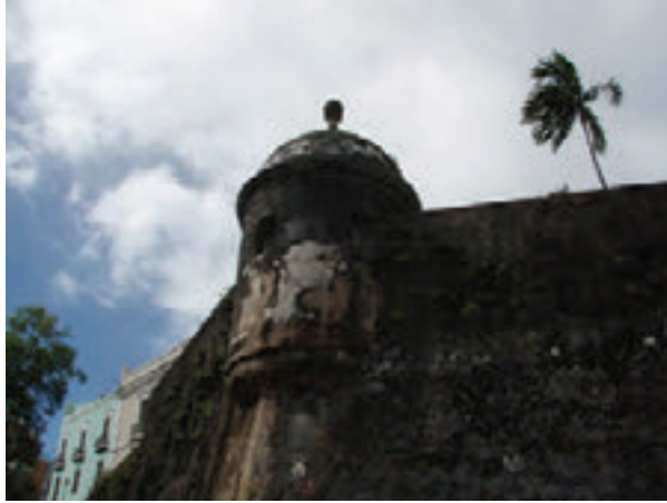
Photo 1: Sentry post with significant lateral cracking across face.
