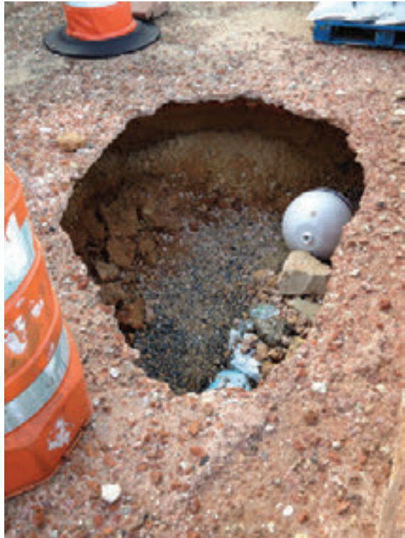
Photo 4: View of void undercutting deck.
