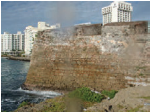
Photo 7: East side erosion and cracking on southeast corner from top.
