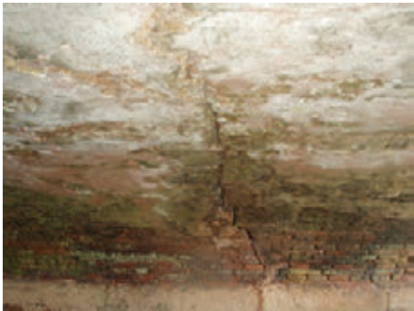
Photo 5: Significant cracking on underside of bridge.
