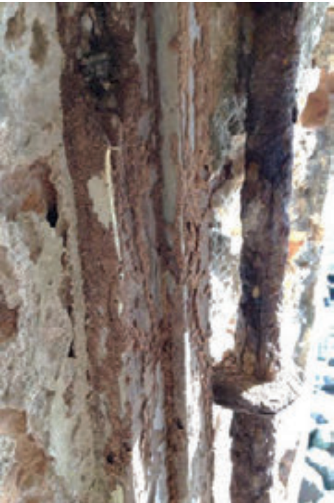
Photo 31: Extensive termite damage to window frame.
