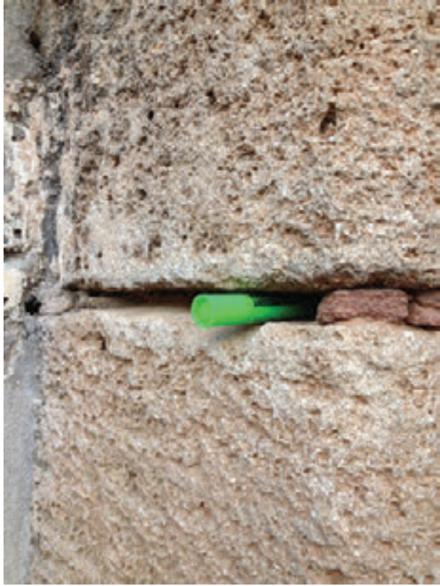
Photo 19: Voids six inches deep into wall.
