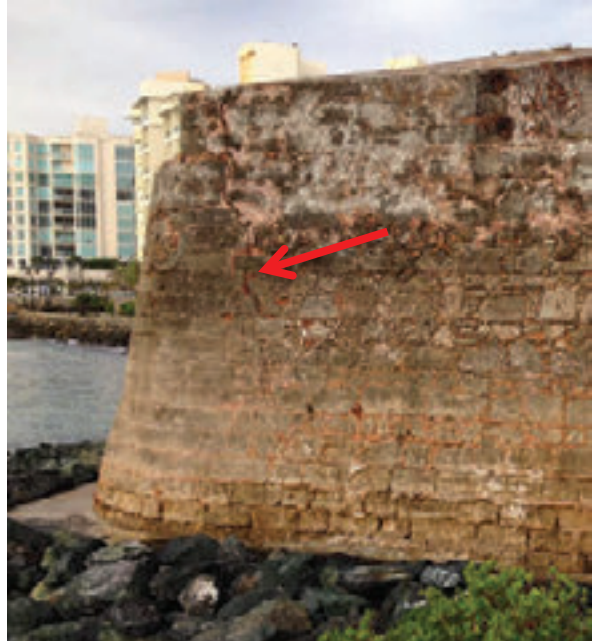
Photo 38: Crack on east exterior wall from foundation to upper escarpment.
