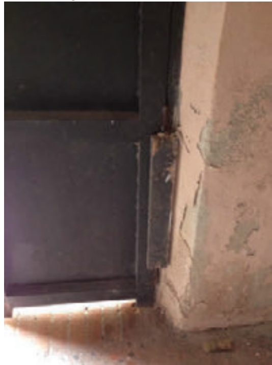
Photo 32: Door held in place by plywood due to broken hinges.
