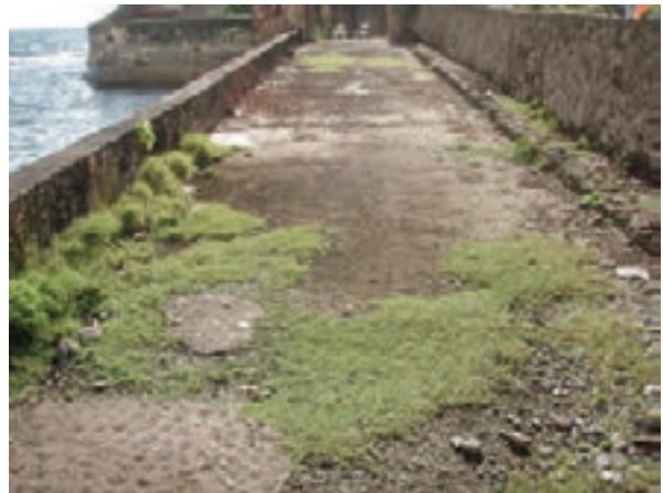
Photo 12: Remove vegetation and inappropriate repairs and resurface bridge.
