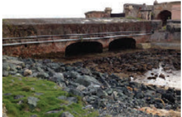
Photo 34: Utilities mounted to the south side of the bridge.
