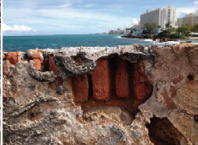
Photo 16: Close up of typical cement and mortar erosion.
