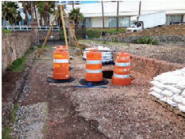
Photo 1: Barricade around void in bridge deck.
