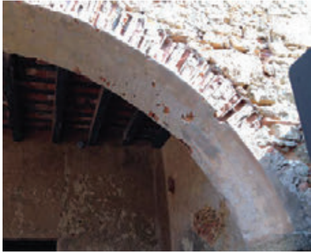
Photo 13: Missing bricks form Portico arch.
