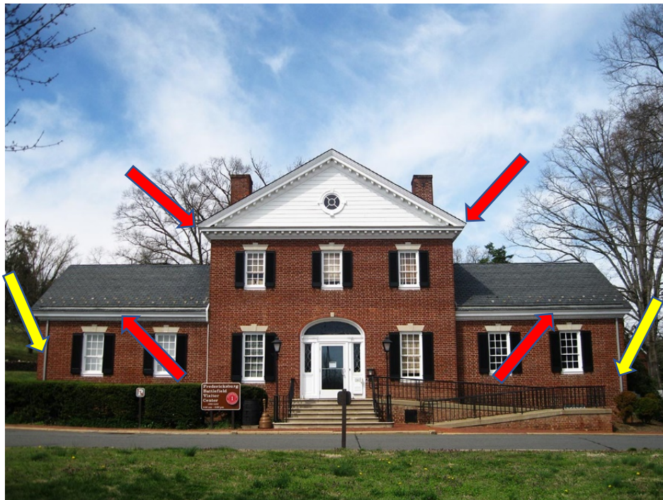
Four exterior gutters will be installed- two on the front of the two wings and two on the sides of the central portion – identified by red arrows. Two downspouts will be installed on the front of the building – one on each wing – identified by the blue arrows.
