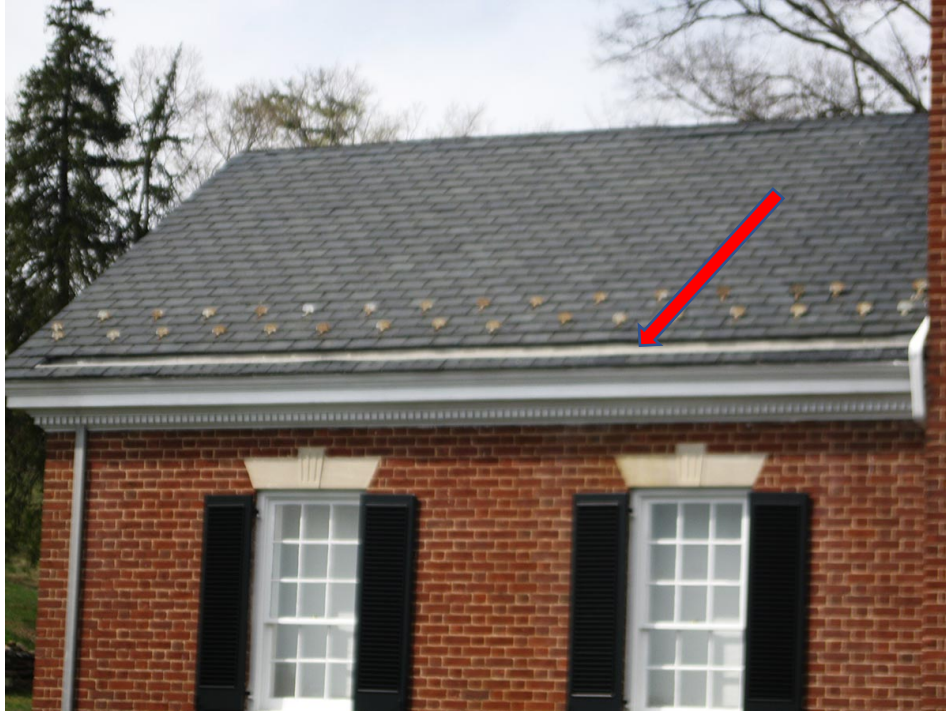
Interior gutters on the Fredericksburg Battlefield Visitor Center. The visible temporary downspouts will be removed, and new exterior gutters and downspouts installed.
