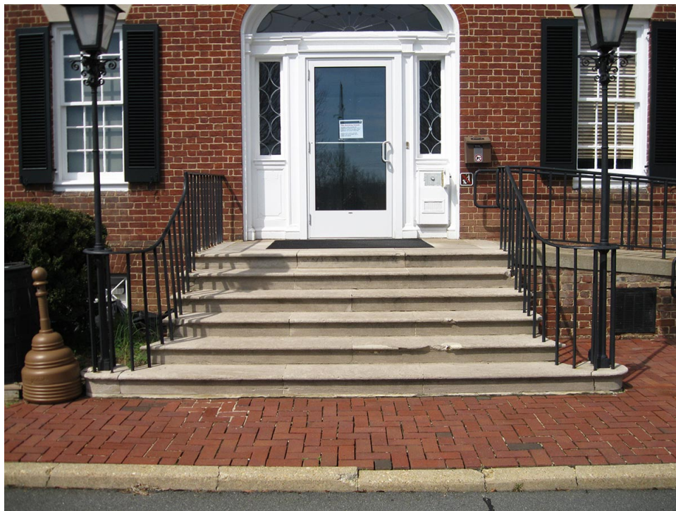
The original 1935-1936 front steps of the Fredericksburg Battlefield Visitor Center. The steps will be removed and replaced. Any damaged material will be replaced with in-kind materials and with in-kind design. To include railings and light poles.
