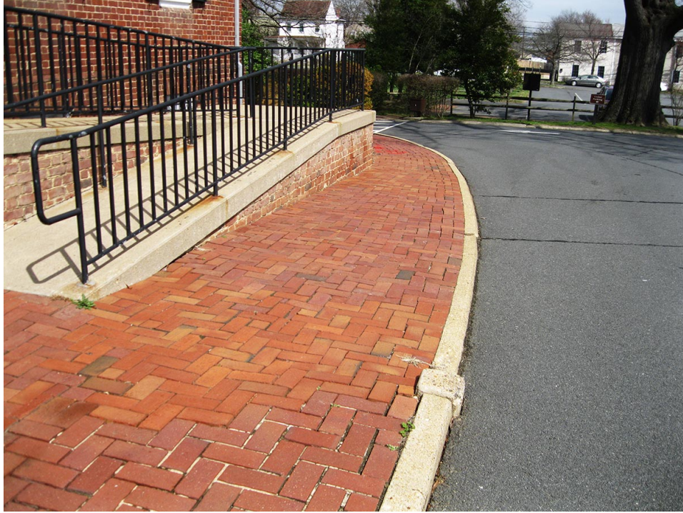
American Disabilities Act (ADA) Ramp on the front of the Fredericksburg Battlefield Visitor Center. The ramp was constructed in 1985. It will be removed and rebuilt, but will be 1-2 feet longer and 1-2 feet wider to comply with more recent ADA requirements.
