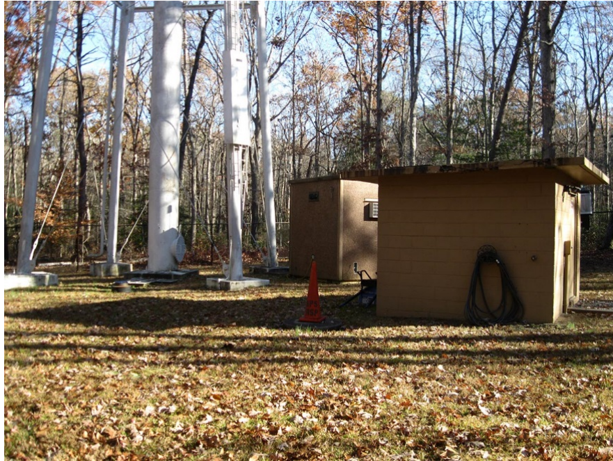
Well house at the base of the Chancellorsville water tower. The orange cone marks the failed well.
