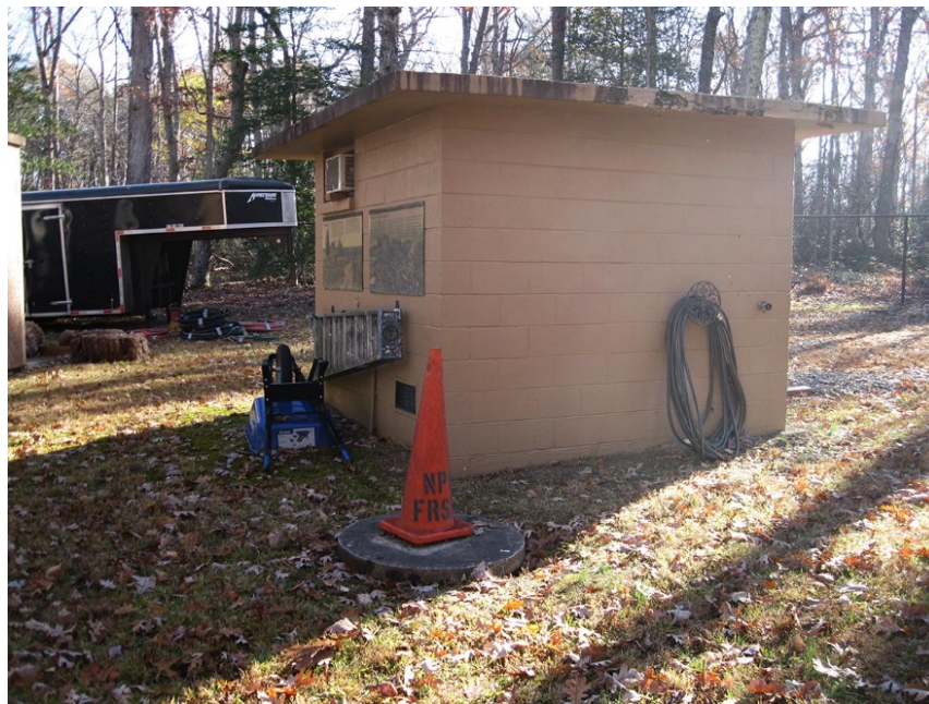
Well house at the base of the Chancellorsville water tower. The orange cone marks the failed well. A new well will be drilled within ten feet of the well house and a supply line run to the building.
