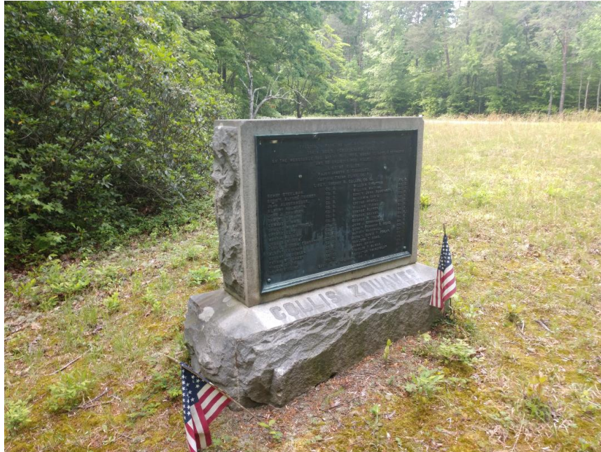
The 114 th PA Monument, with Route 3 in the background. Note the stains on both the stones and metal tablet, a result of lack of safe access for maintenance crews to clean the monument and the encroaching forest cover.
