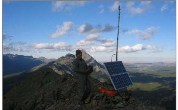
*Example of a temporary, or scene-of-action, radio repeater. NPS photo.*
