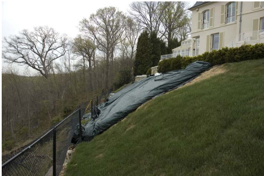
Existing Site Conditions - Wall failure/landslide area (NPS photo, April 2007)
