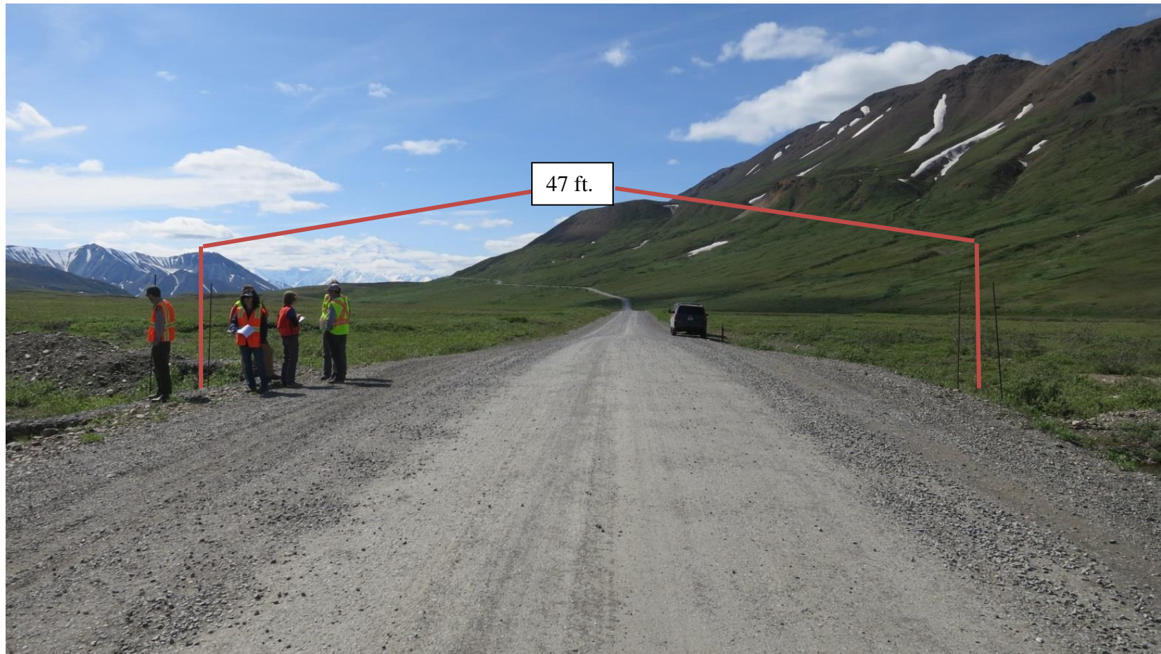
Figure 7- 47 ft. wide road width at Krier's Creek looking west (from steam pipe to steam pipe) (NPS Photo, July 17 th , 2018).
