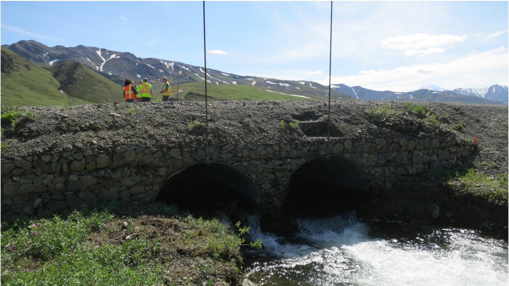
Figure 9- Krier's Creek existing north (downstream) side gabion basket wall (looking SW) Note drop in elevation from culvert to pool making fish passage impossible. (NPS Photo, July 17 th 2018).
