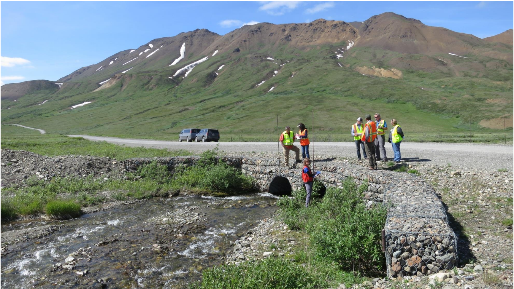
Figure 8-Krier's Creek existing south (upstream) side gabion basket wing walls and culverts (looking NW) (NPS Photo, July 17 th 2018).
