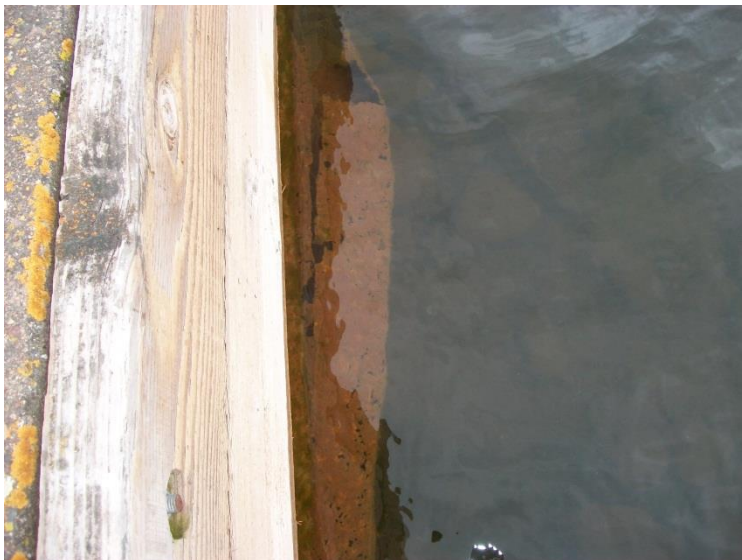
Figure 4. Degradation of Siskiwit Dock cribbing. The binwall panel has rusted and is falling away from dock.
