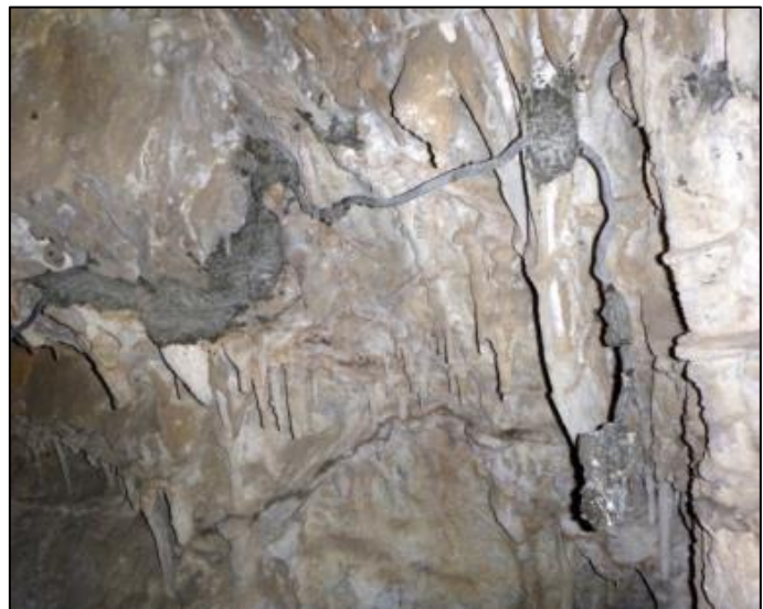
Figure 40. Old lighting systems damaged cave formations and applied excessive grout that is now peeling away.
