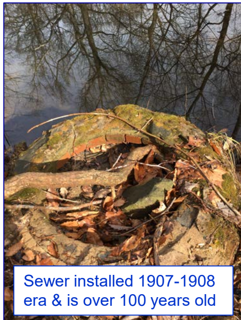
Manhole near stream and exposed sanitary sewer pipe
