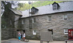
Difficult to access rest rooms
