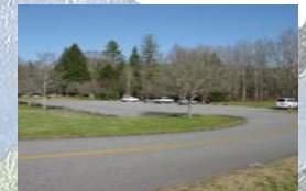
Poor vehicle access and parking
