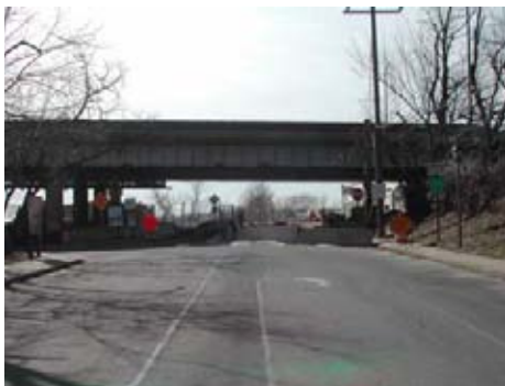
Looking south at existing bridge from Royal Street
