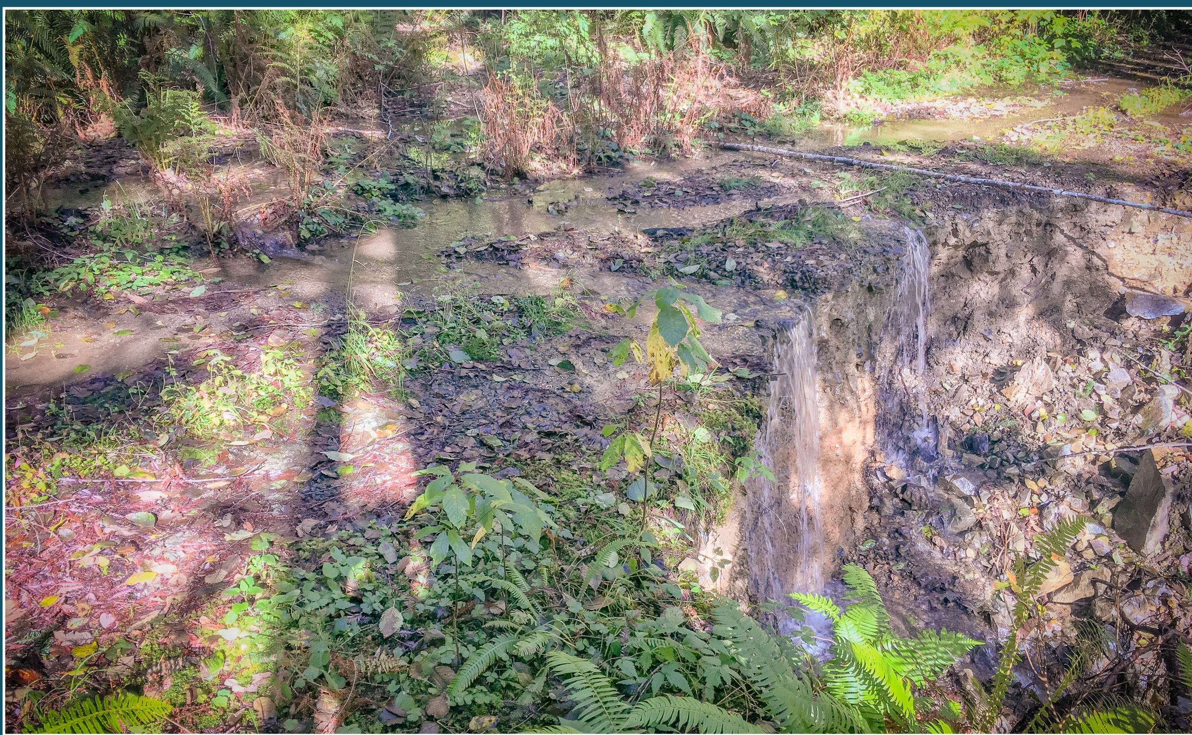
A remaining logging road slowly erodes away, putting sediment into streams.
