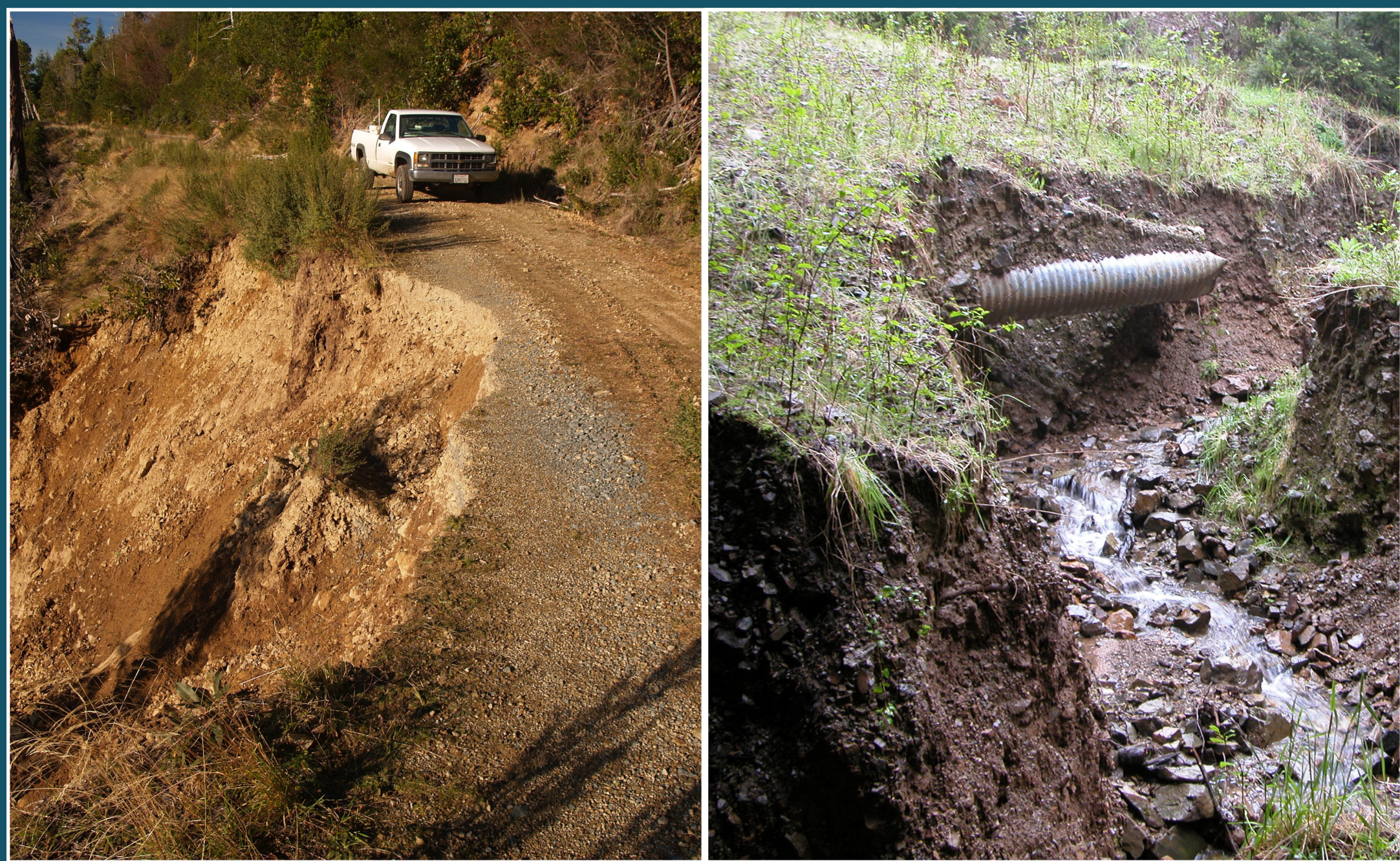
Abandoned roads are not usable by vehicles or heavy equipment. Because they have not been maintained, they erode during storm events and contribute large inputs of sediment to the streams. These roads will be upgraded for forest restoration access, then removed when restoration in the area is completed.
