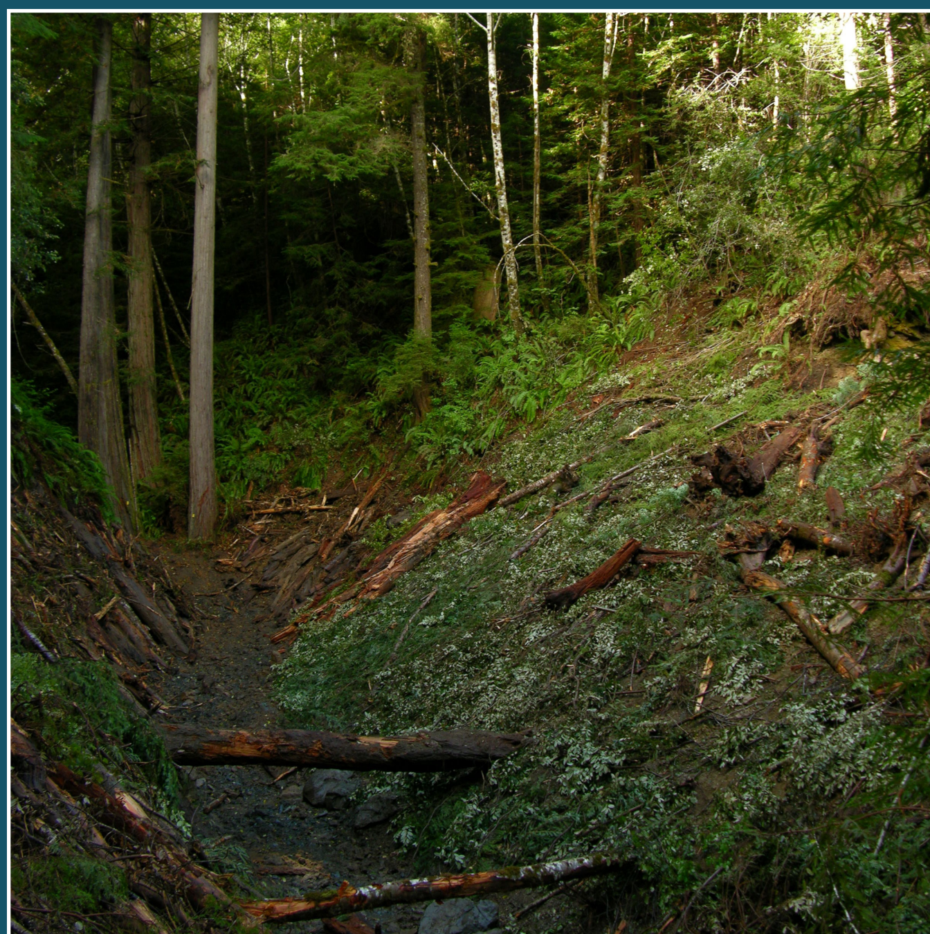
The same stream crossing after treatment; the stream banks are shaped to the existing hillslope above and below the removed road. Vegetation and logs that were removed from the road prism are spread over the surface as mulch.
