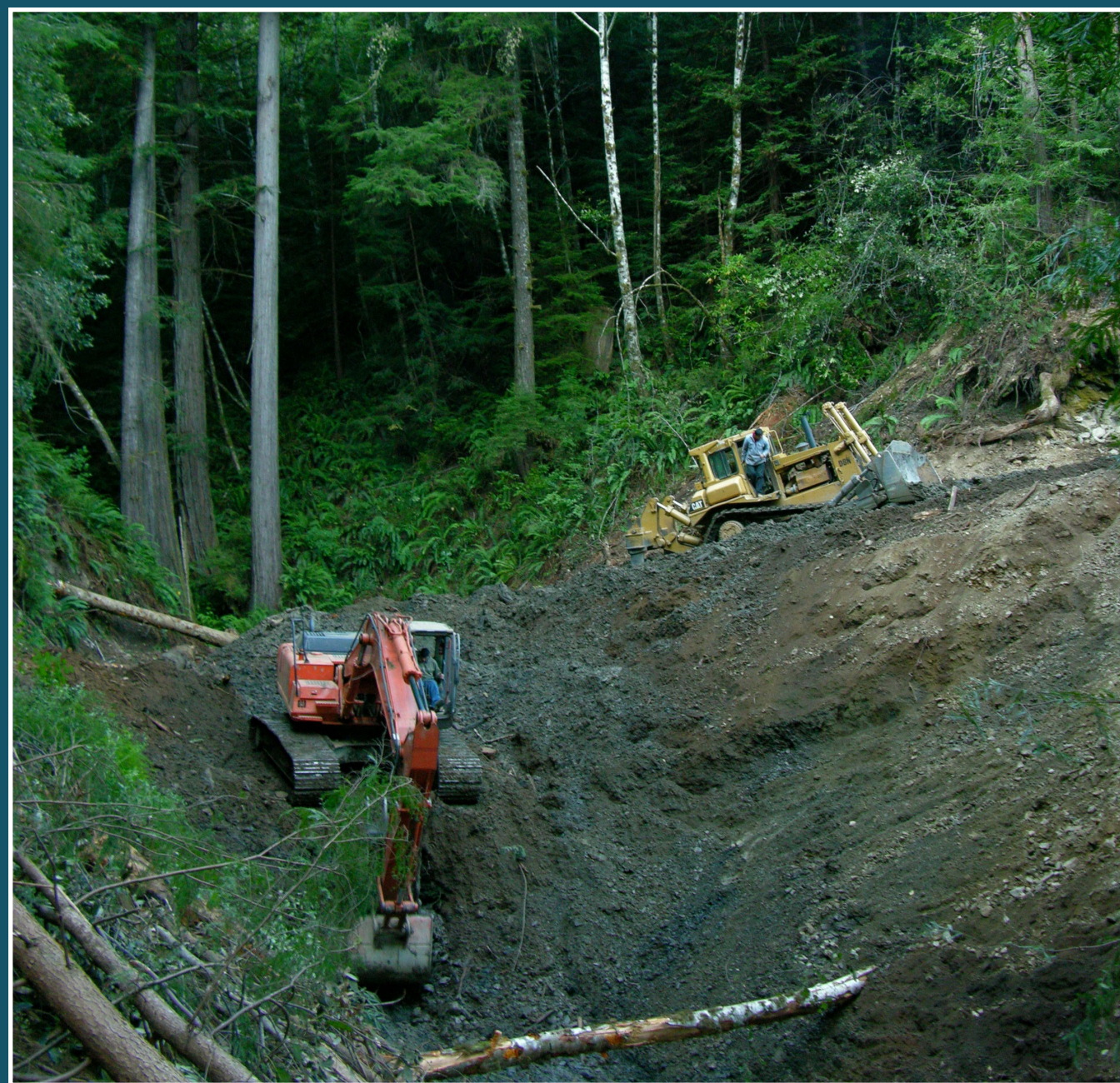
An excavator removes a stream crossing by digging down to the original buried stream channel. The fill is placed on the road, where a bulldozer pushes it out to an adjacent cutbench to be stabilized and recontoured into the hillslope.
