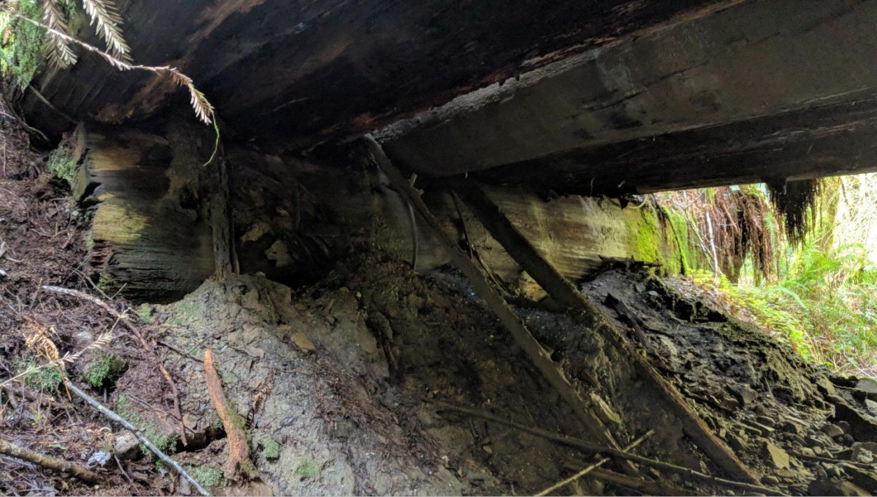
Failing south abutment of log stringer bridge: one log 30' long & 6' in diameter
