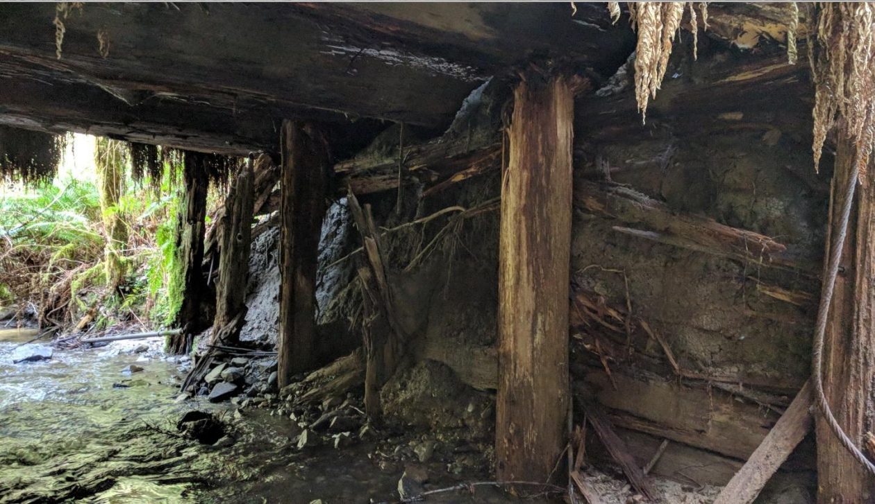
Failing north abutment of log stringer bridge: two logs 15-20' long & 4' in diameter
