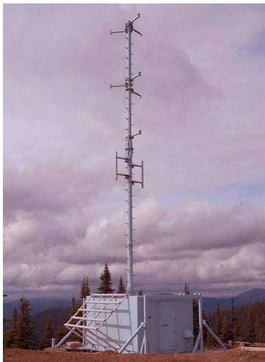
Figure 5, Example Radio Tower (self supporting 100 ft lattice tower of the type proposed for CC Hill, however the CC Hill tower would be 150 ft tall and would not be red/white striped)
