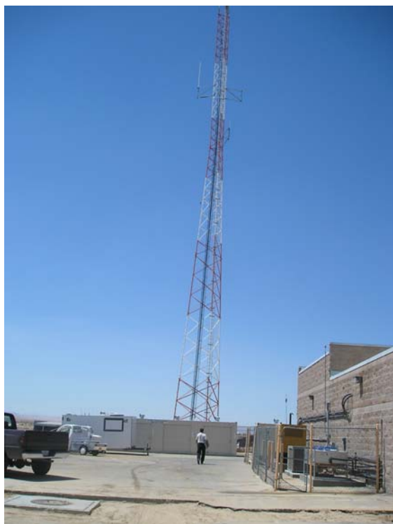
Figure 5, Example Radio Tower (self supporting 100 ft lattice tower of the type proposed for CC Hill, however the CC Hill tower would be 150 ft tall and would not be red/white striped)
