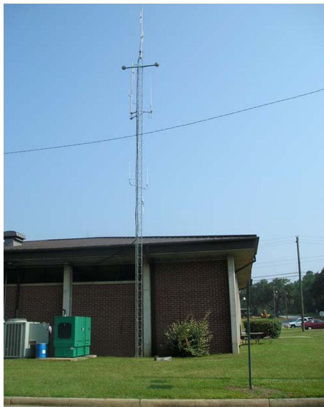
Figure 4, Example Radio Tower (self supporting 60 ft. lattice tower of the type and size proposed for Desert View, Hopi Fire Tower, and Grand Canyon EMS)
