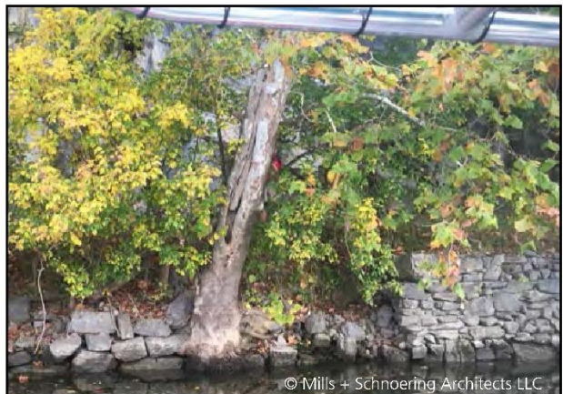
2f. Stone wall collapse
