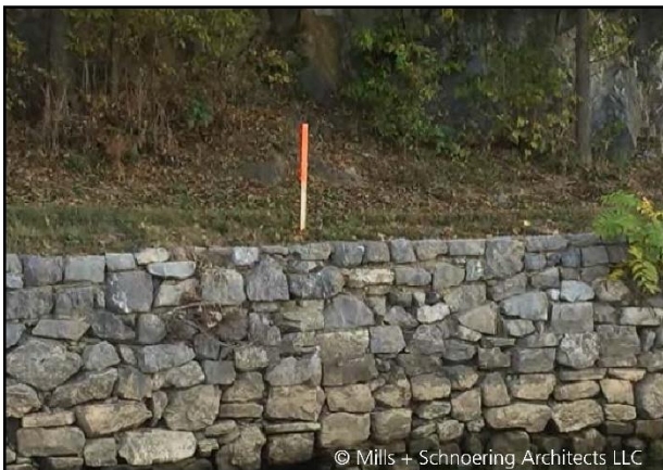
2e. Undermining along the base of the stone wall
