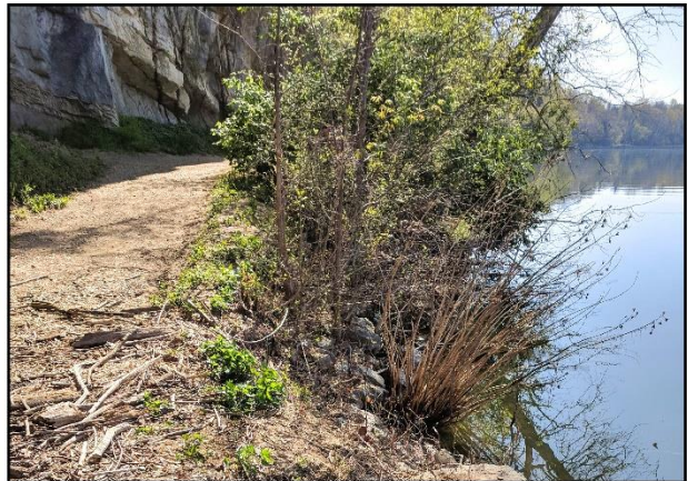
2d. Vegetation growing out of the stone wall
