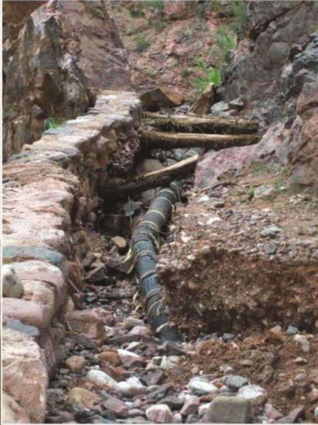
Photos of Exposed Pipeline
