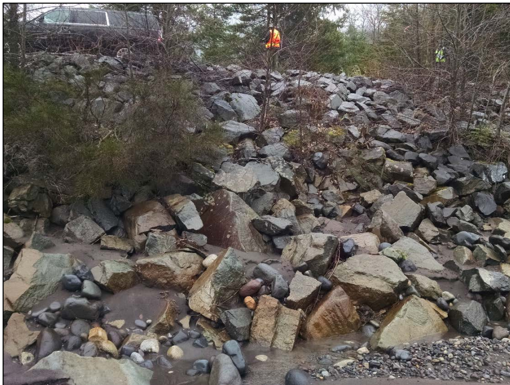
Photograph 4: Site 2 damage. Voids in face and slope toe.
