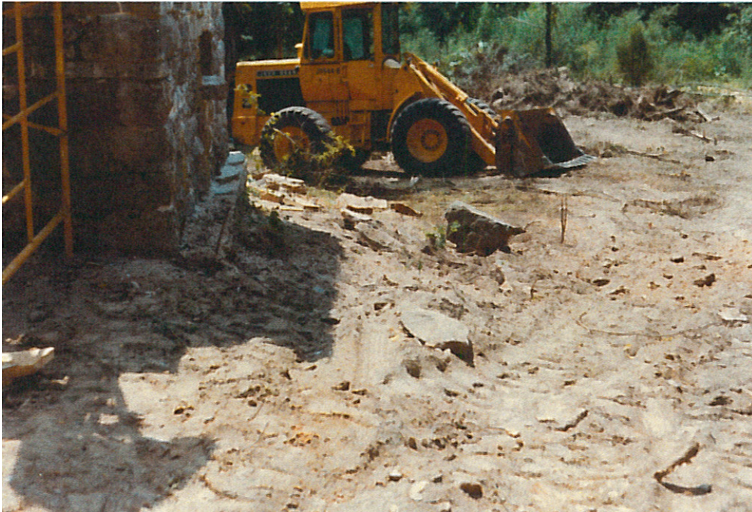
Figure 2-64. Stabilization of the Rush Smelter included earthwork around the base of the smelter as part of the overall stabilization effort, c 1985. (BUFF Archives)
