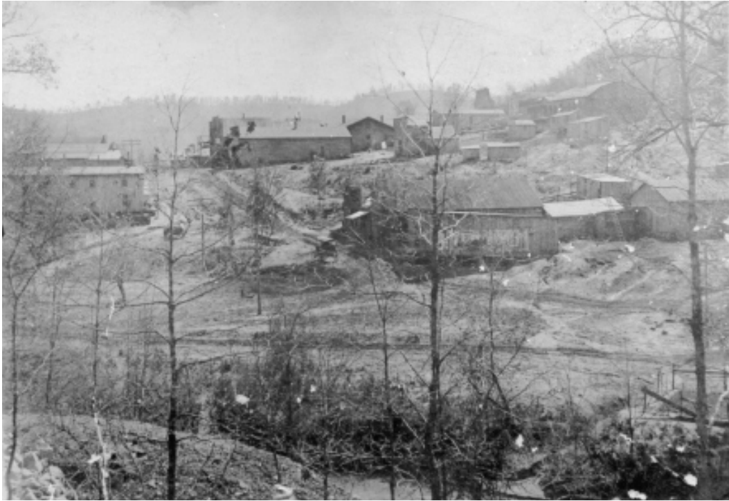
Figure 3-4. New Town as it appeared c 1916 from the north bank of Rush Creek. The development of New Town was spurred by mining expansion during World War I that led to construction of Edith Mine (M12) and a new mill at Yellow Rose Mine (M7) (uphill on right). Today only a few ruins of New Town are visible above grade. Below grade resources associated with these mine complexes likely exist as they do throughout the study area. (Buffalo National River: Dorthea Shipman Collection)
