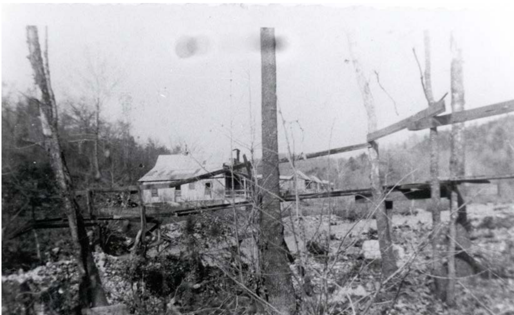
Figure 3-32. Footbridge across Rush Creek, Taylor-Medley General Store behind, date unknown. (BUFF Archives)
