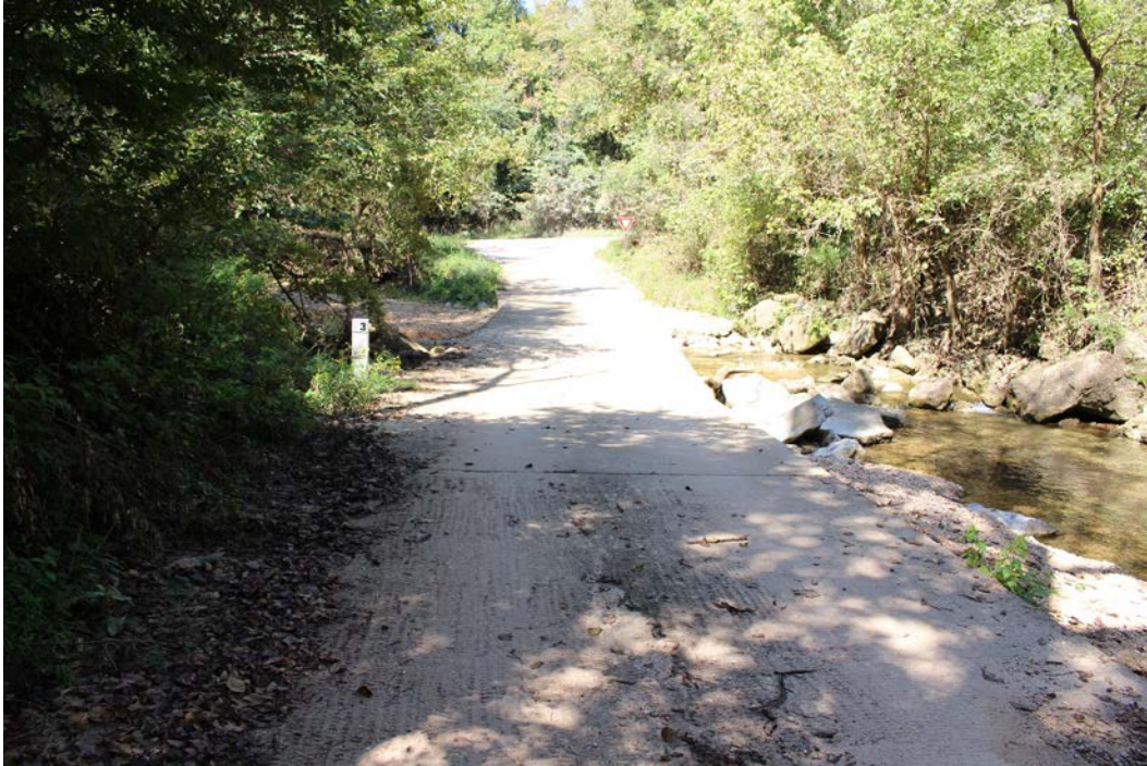
Figure 3-23. Campground Road concrete water crossing at Rush Creek. Campground Road is part of the original route to New Town, Yellow Rose Mine Complex (M7), and Edith Mine Complex (M12), established in the early 1900s. (Mundus Bishop 2017)
