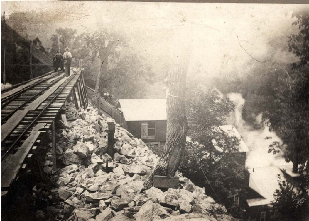
Figure 3-31. Gravity-fed tramways shipped ore from mines to mills. The exact route of these tramways is unknown, except near Morning Star Mill, where the tramway piers are extant, date unknown. (BUFF Archives)
