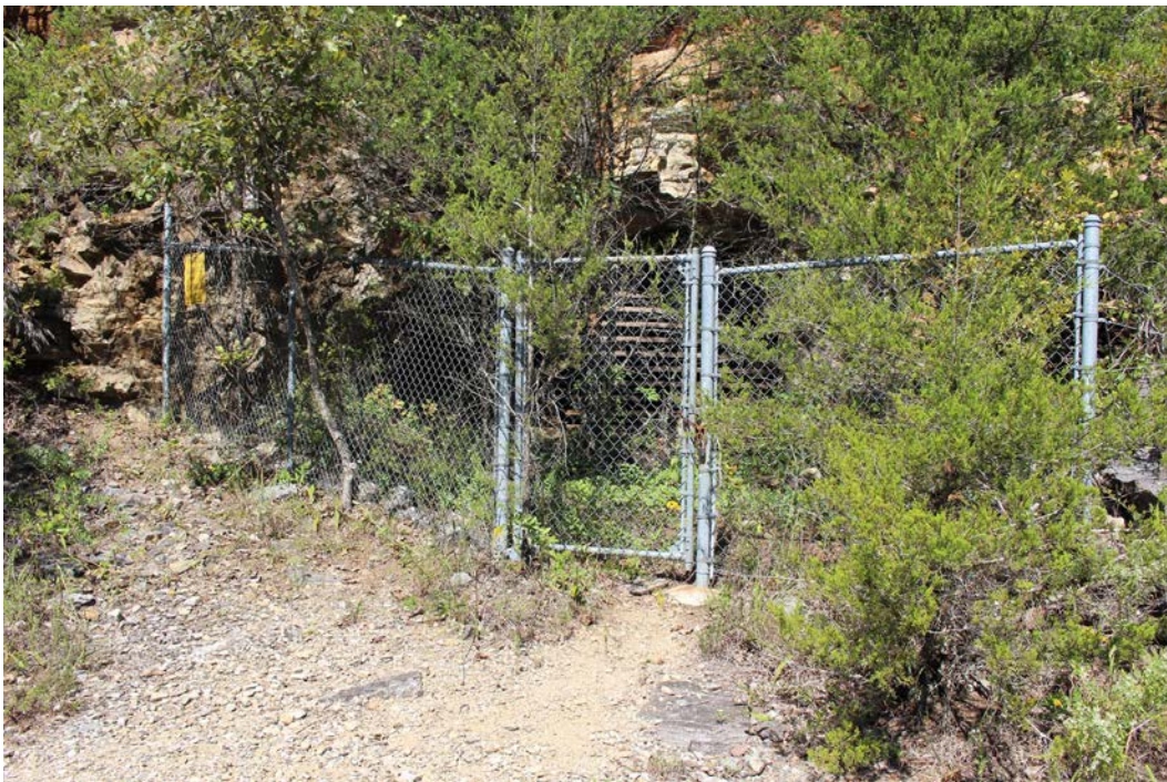
Figure 3-38. Chainlink fencing has been installed across most mine entrances. This fencing distracts from the historic character. (Mundus Bishop 2017)
