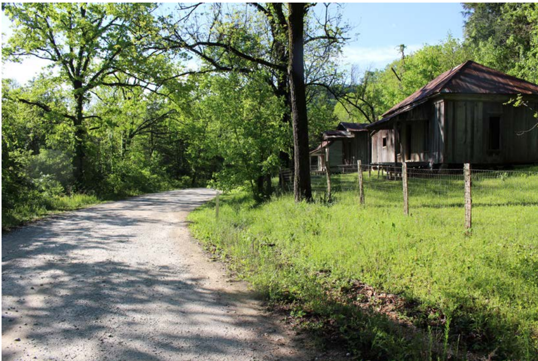
Figure 3-18. Rush Road at House Row. The road retains its historic alignment but has been widened and resurfaced since the period of significance. (Mundus Bishop 2017)
