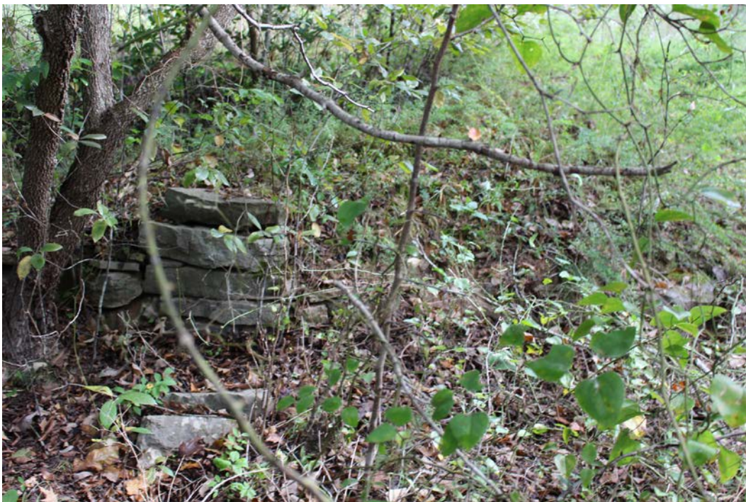
Figure 3-102. Stone retaining wall at Chase and Mulholland Store. (Mundus Bishop 2017)
