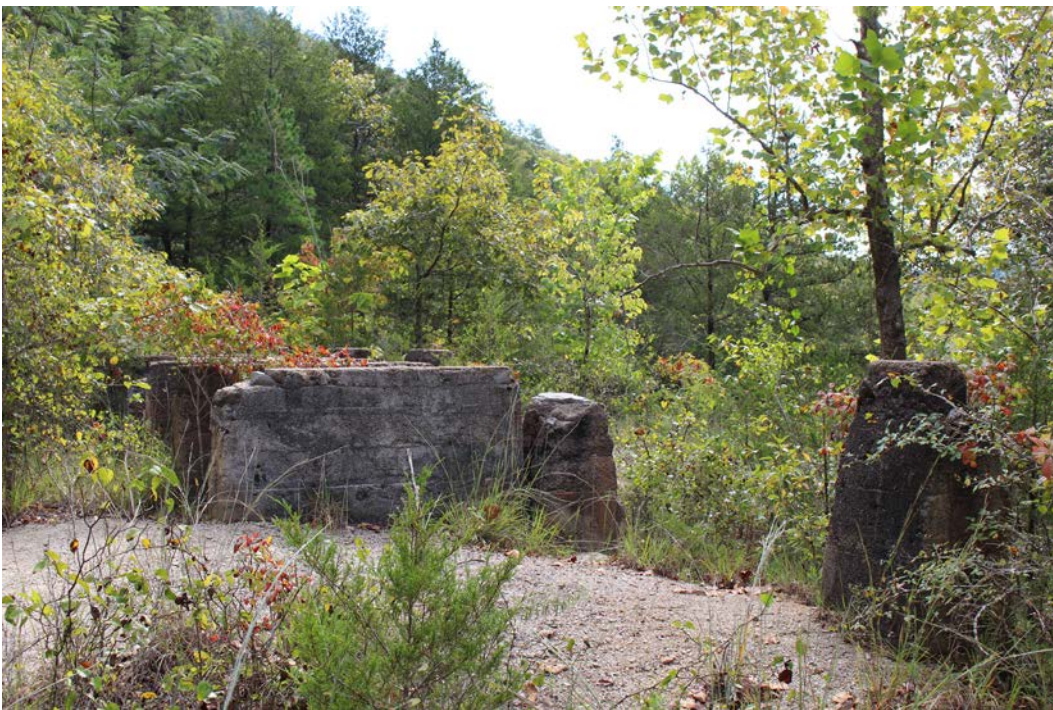
Figure 3-94. Morning Star Mill ruins include a series of concrete and stone piers, a stone retaining wall at the northern slope, a concrete platform for the engine, and a stone and brick boiler room. The mill is set on a level terrace above the remainder of Morning Star Hotel, Mill, and Mine Community. (Mundus Bishop 2017)
