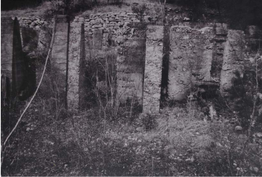
Figure 3-122. Morning Star Mill retention basin concrete spillway, c 1980s. (BUFF Archives)
