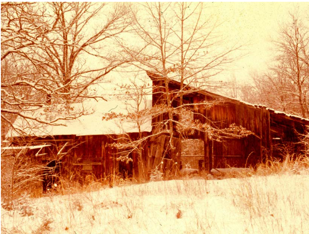
Figure 3-109. Rush Blacksmith Shop and Warehouse, date unknown. (S. Rogers, BUFF Archives)
