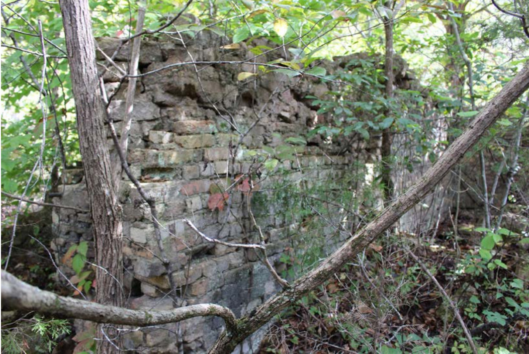
Figure 3-116. Morning Star Mill ruins Boiler Room. (Mundus Bishop 2017)
