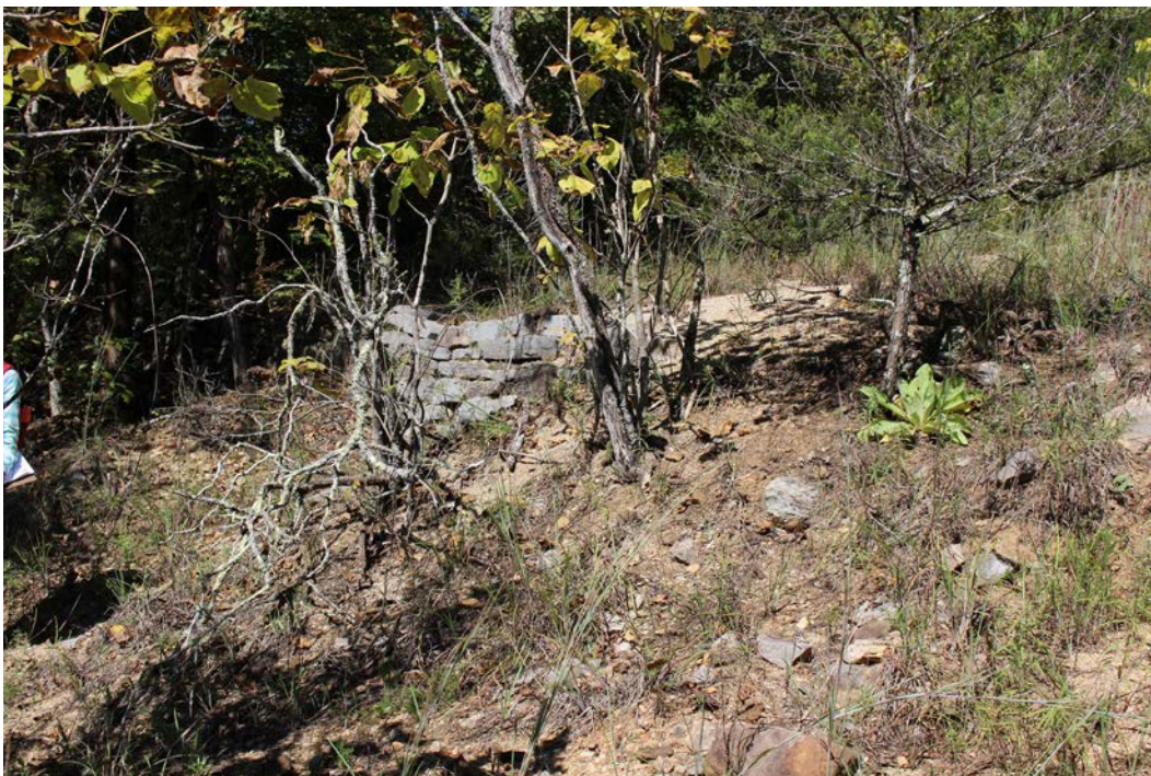
Figure 3-115. Morning Star Mill Stone Retaining Wall, near Boiler Room. (Mundus Bishop 2017)
