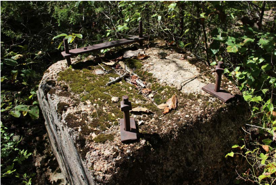
Figure 3-121. Concrete engine mount at Morning Star Mill ruins. (Mundus Bishop 2017)
