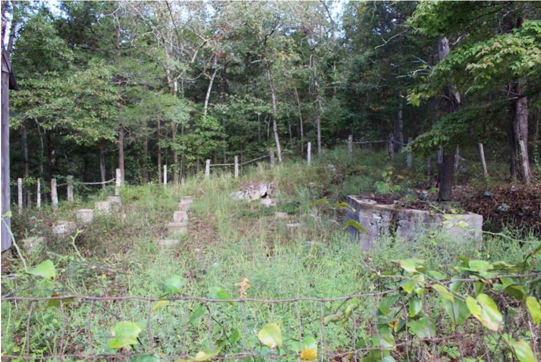
Figure 3-111. Warehouse piers and foundations. (Mundus Bishop 2017)
