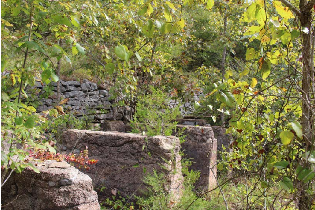
Figure 3-112. Stone and concrete piers, and stone retaining wall (rear) at Morning Star Mill ruins. (Mundus Bishop 2017)
