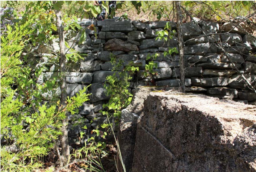
Figure 3-117. Stone retaining wall and concrete pier. (Mundus Bishop 2017)
