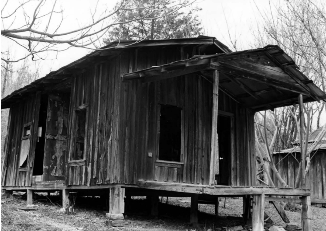
Figure 3-138. Wash House, 1984. (S. Rogers, BUFF Archives)
