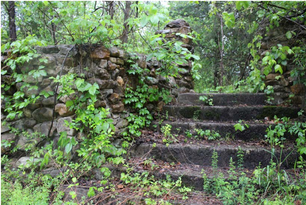
Figure 3-156. Hicks Wall, cobblestone columns and concrete stairs. (Mundus Bishop 2017)
