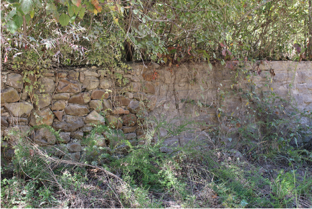
Figure 6-18. Repairs will preserve the Hicks Wall's variety of stone construction techniques (cobblestone and coursed ashlar stone). (Mundus Bishop, 2017)
