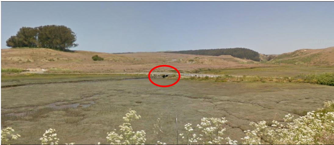
Figure 11: View of Double Culverts Looking North from Ranch N Road
