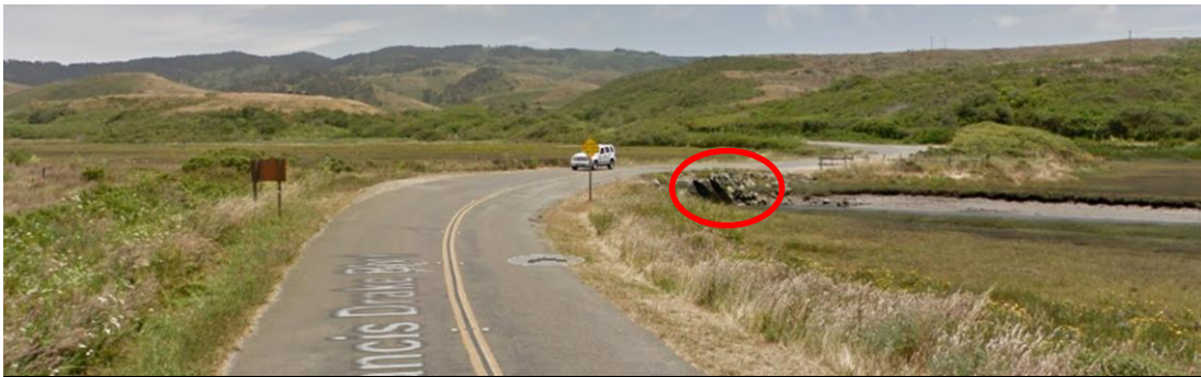
Figure 10: View of Double Culverts Looking Northeast from Sir Francis Drake Boulevard
