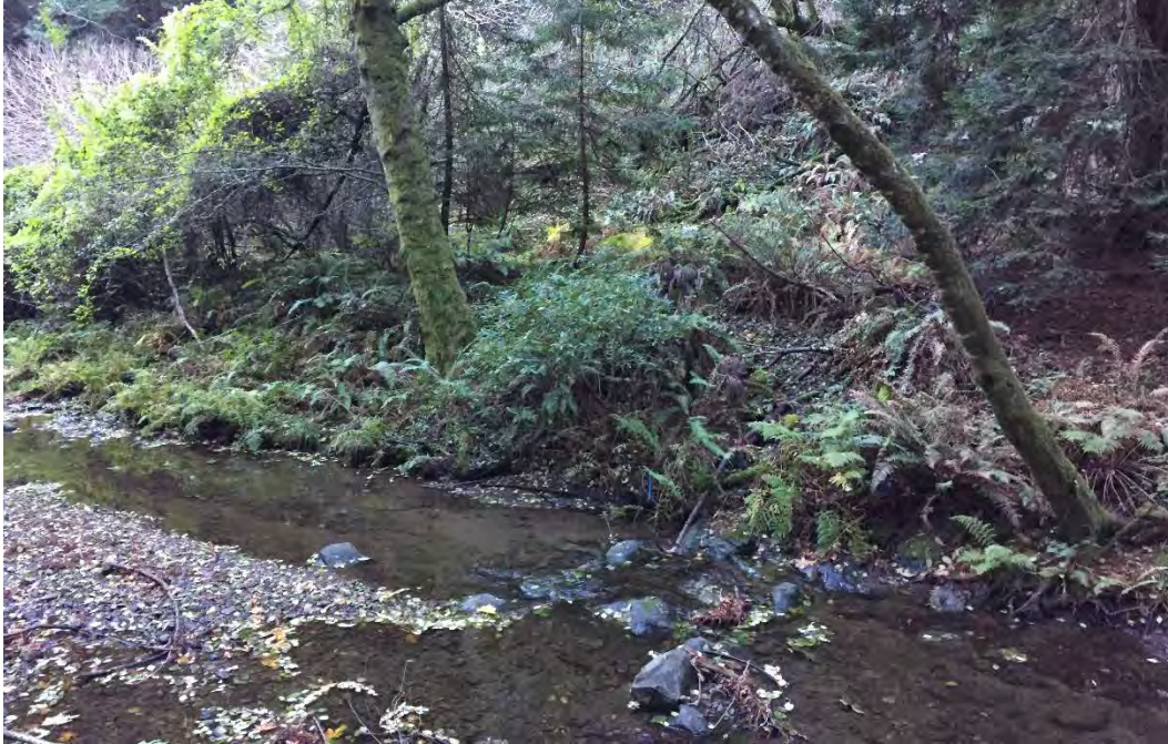
Figure 7. Center-west stretch of Section R1A, view south-southwest from creek bed, showing riprap of medium-sized rocks in good condition beneath vegetation and with trees growing from some areas
