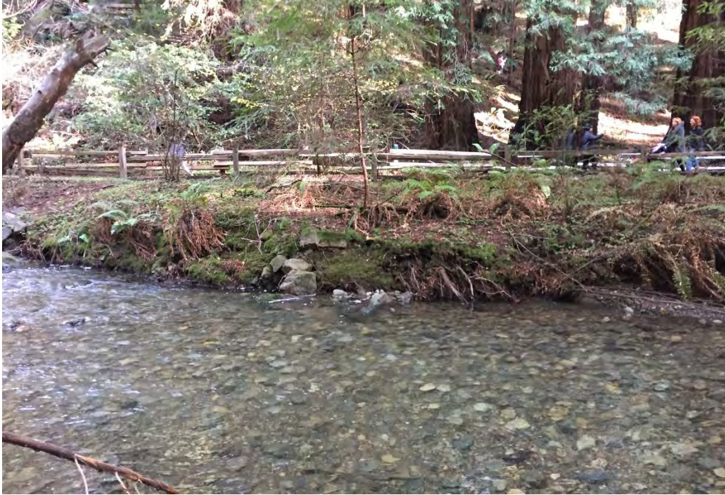
Figure 33. Section L3 seen from right bank, camera facing northeast, showing occasional rocks beneath moss, ferns, and other vegetation. The shape of the bank suggests riprap is in poor condition
