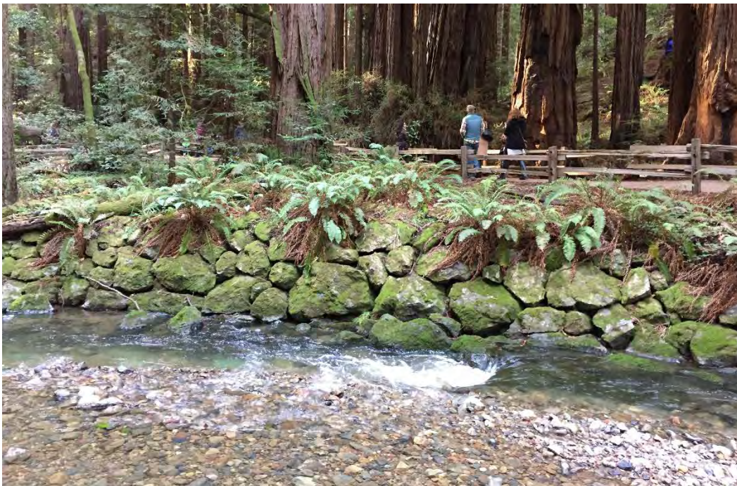
Figure 43. View of Section R4, camera facing southwest, large- and medium-sized rocks in excellent condition below fern growth
