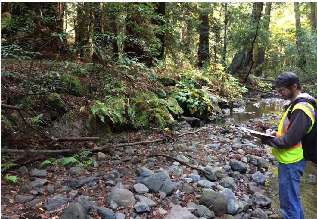
Figure 76. Center stretch, view east from creek bed, showing ferns and small tree grown atop riprap in good condition
