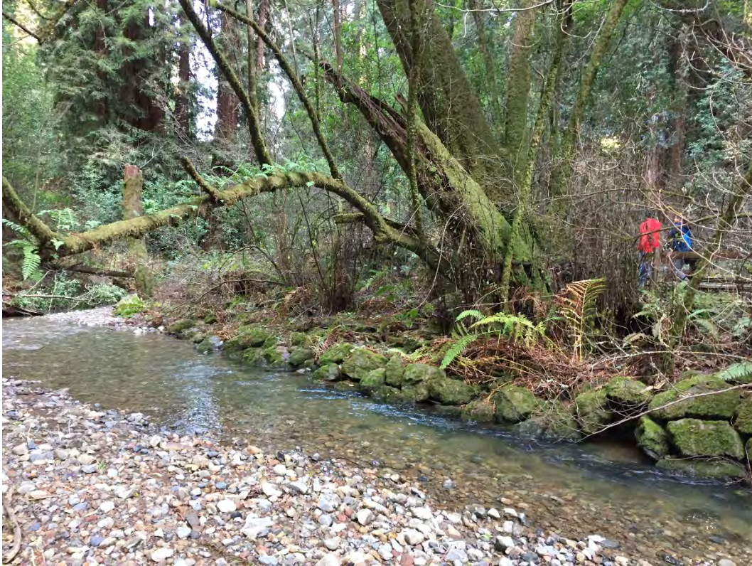
Figure 26. Section R3A from left bank, camera facing east, showing east stretch with 2-4 course riprap in excellent condition
