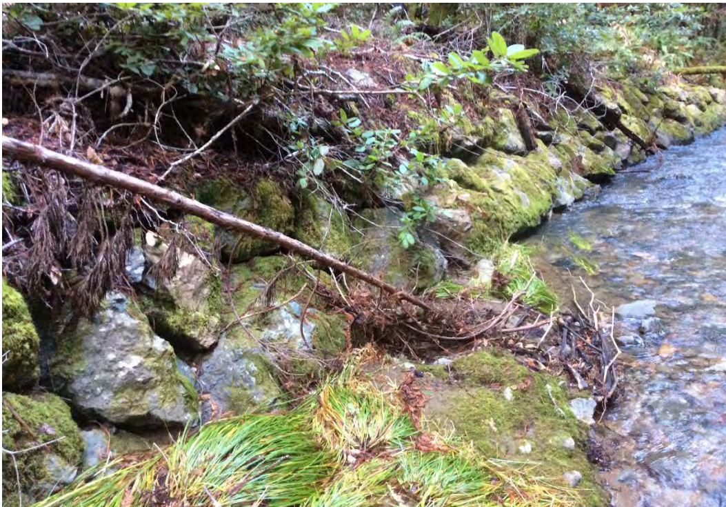
Figure 97. Center stretch of Section L12, view west from creek bed, showing riprap tightly-stacked and in excellent condition
