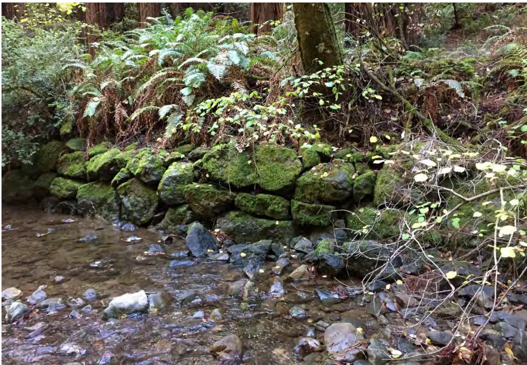
Figure 93. Detail, west stretch view south, showing riprap in excellent condition
