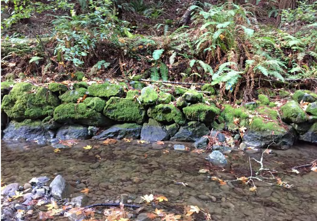
Figure 81. Detail, west stretch, showing riprap in excellent condition with ferns above
