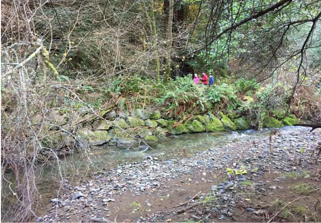
Figure 18. Section R2 viewed from left bank, camera facing southwest, showing tightly placed medium-sized rocks in good condition
