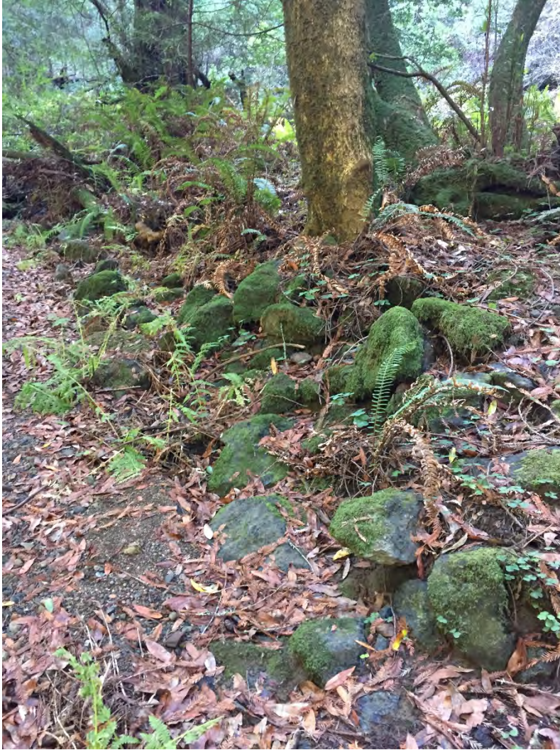
Figure 37. Detail, Section R4, view south, showing riprap in fair condition with ferns and a tree growing out of it
