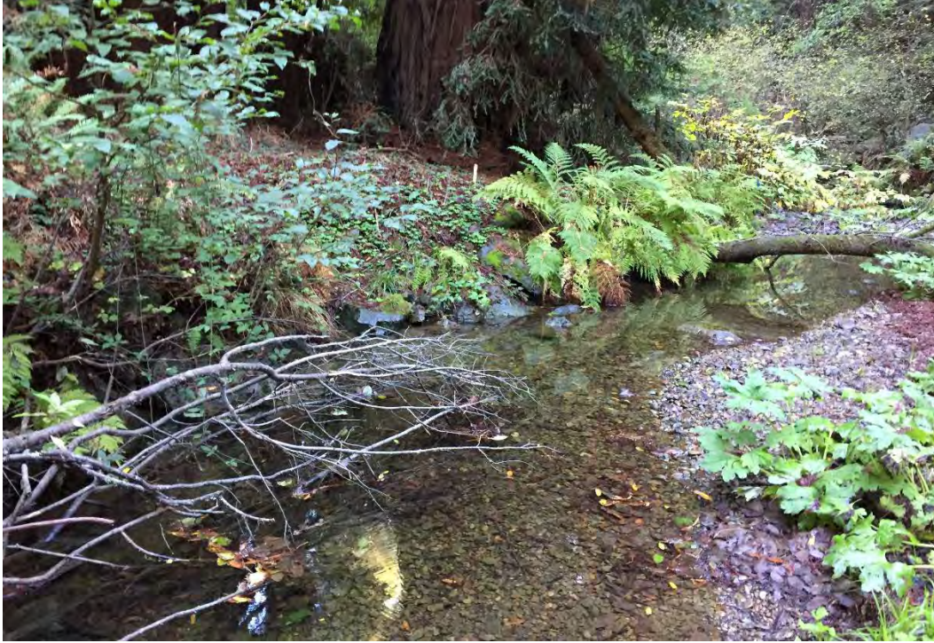
Figure 23. Poor condition downstream stretch of Section L2, view east from right bank, showing deteriorating riprap with woody debris, ferns, and other vegetation
