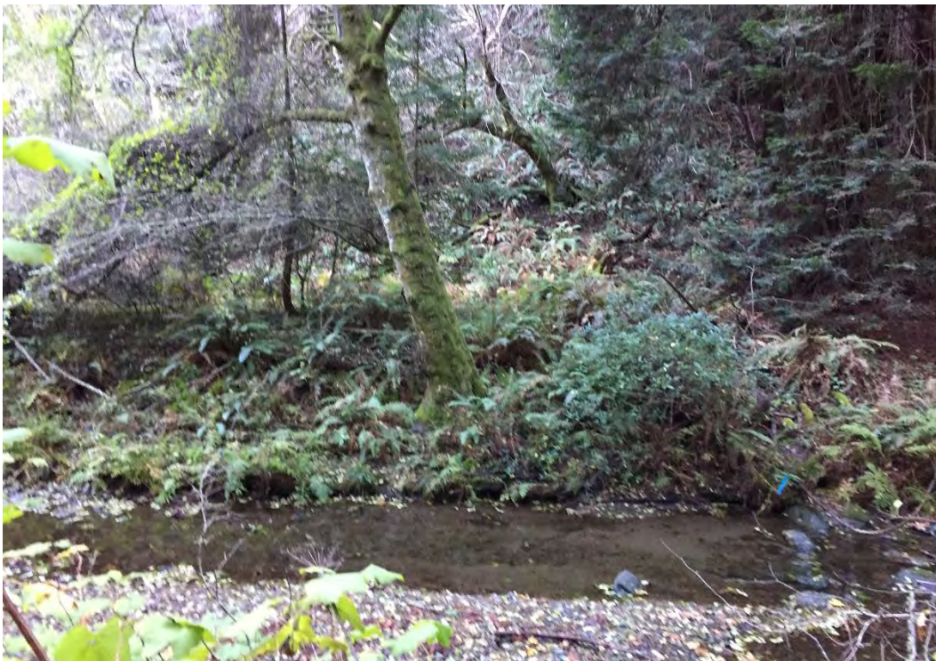
Figure 8. Center-west stretch of Section R1A, view south from creek bed, showing riprap in good condition beneath vegetation and with trees growing from some areas
