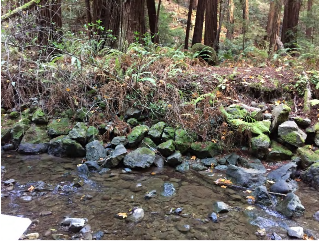
Figure 85. West stretch, view north from creek bed, showing riprap in fair-poor condition with ferns partially obscuring
