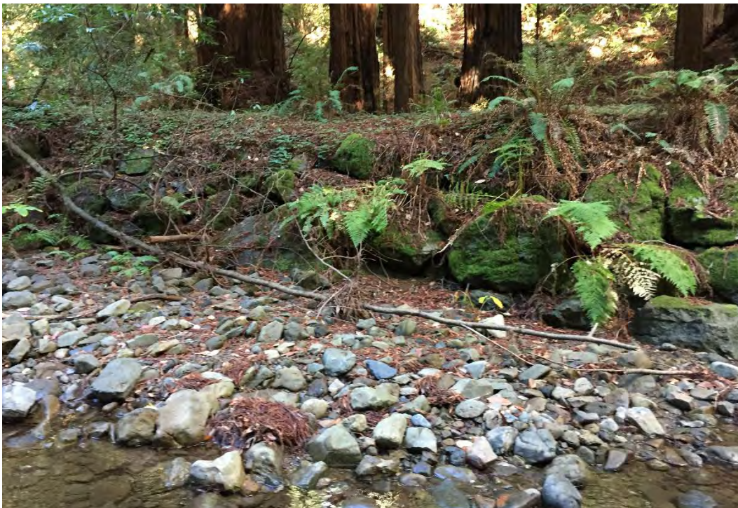
Figure 78. East end showing some displaced boulders with most riprap in good condition beneath light vegetation growth
