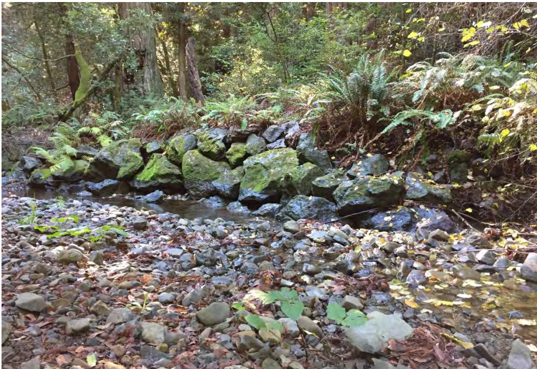
Figure 52. North stretch of Section R6, view west showing riprap in very good condition with small areas of deteriorated or obscured by vegetation at either end
