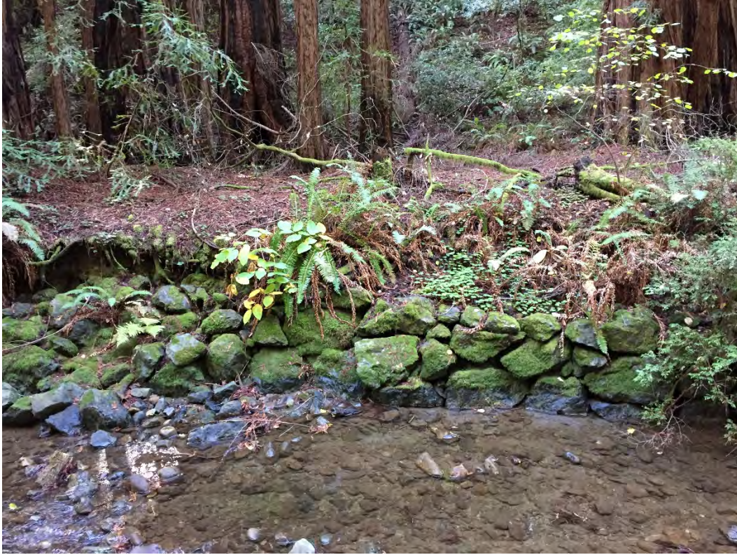
Figure 94. Detail, east stretch view southeast, showing riprap excellent condition with small collapsed area left of frame and ferns growing above
