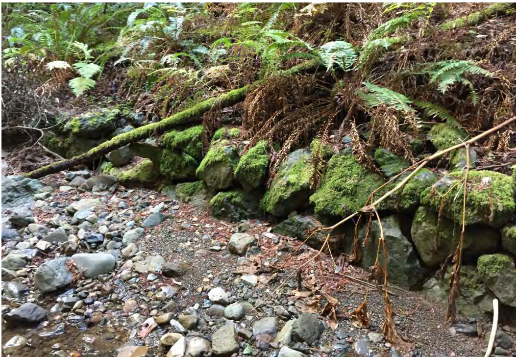
Figure 72. Detail, northwest stretch, showing 2-3 courses of tightly stacked boulders of variable size with ferns and small amounts of woody debris
