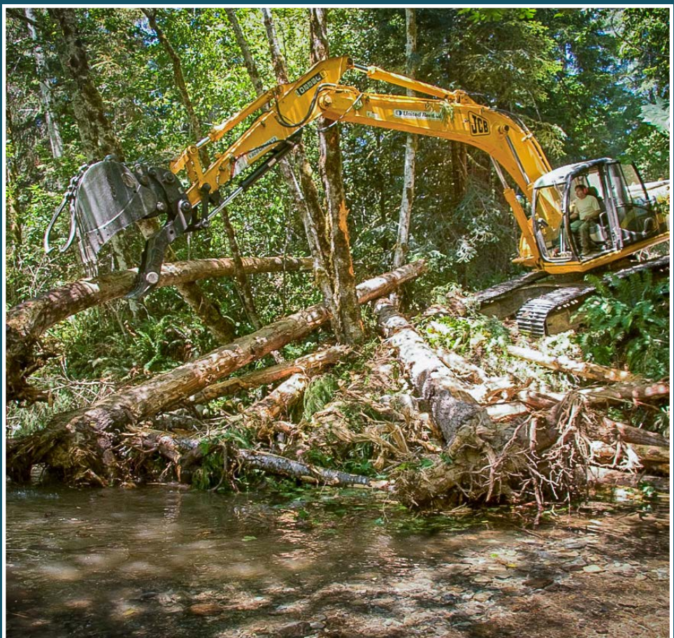
An excavator places large wood into an aquatic habitat structure in Mill Creek. Large wood pieces are interlocked with existing trees on the stream bank to secure the structure.
