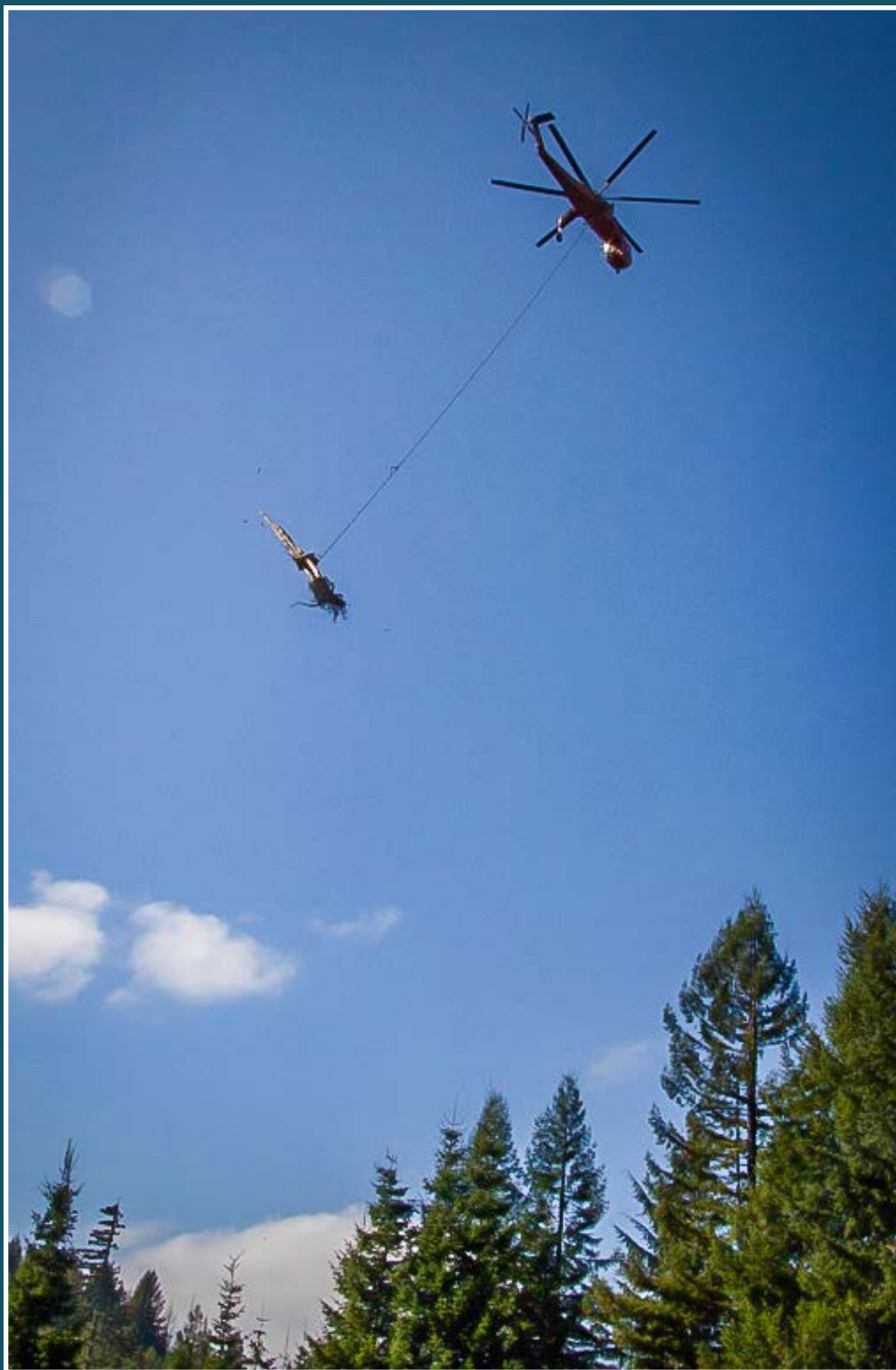
A helicopter transports and places a piece of large wood that will augment previously constructed structures in Mill Creek watershed.
